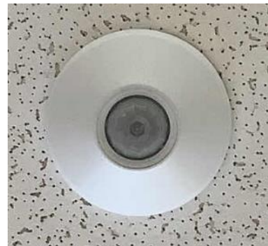
Ceiling Mounted Occupancy Sensor
