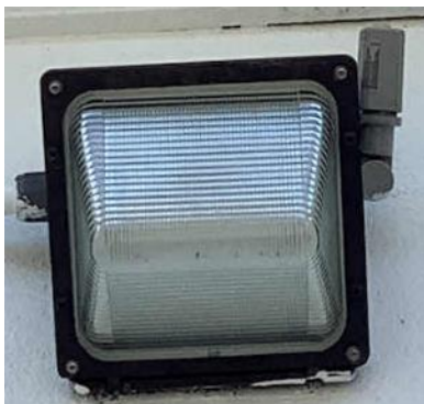
LED Wall Pack with Photocell
