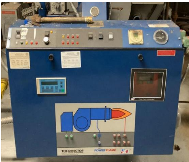
Forced Draft Combustion Burner
