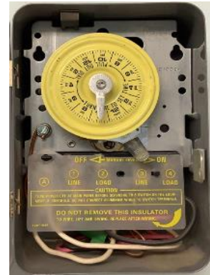
Timeclock for Exterior Lights
