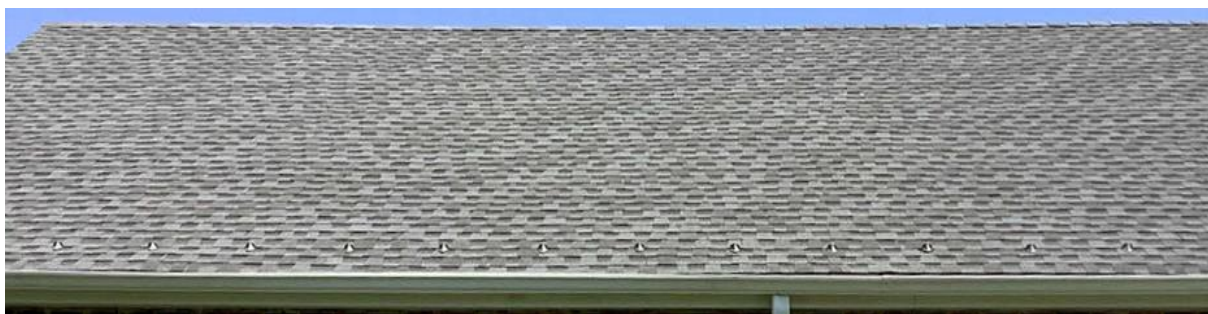
Pitched Roof with Asphalt Shingles
