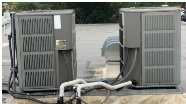
Split AC System Condensing Units
