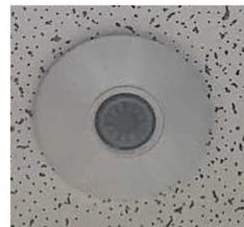
2x4 LED Ambient Pannel, CFL Biaxial Plug-in Lamp, LED Exit Sign, & Ceiling Mounted Occupancy Sensor
