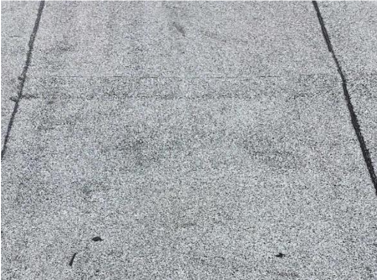
Built-up Asphalt Roof
