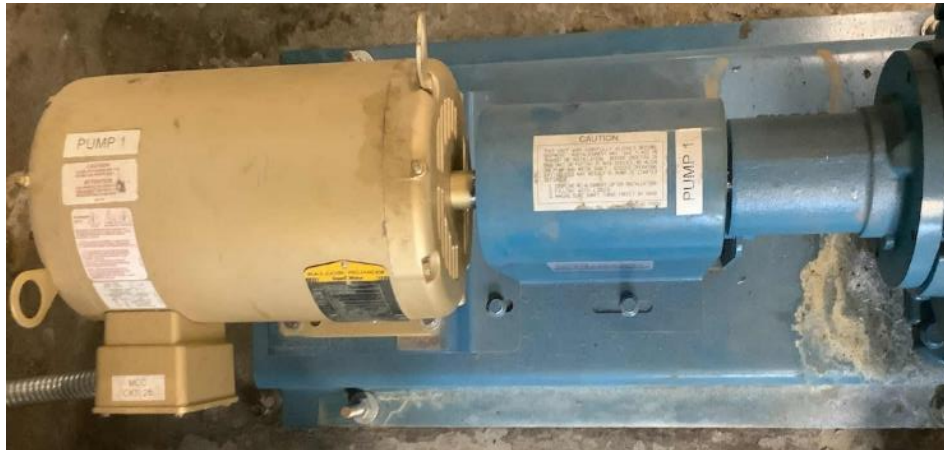
Heating Hot Water Pump
