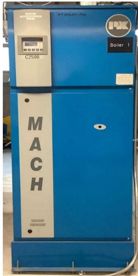
Condensing Hot Water Boiler
