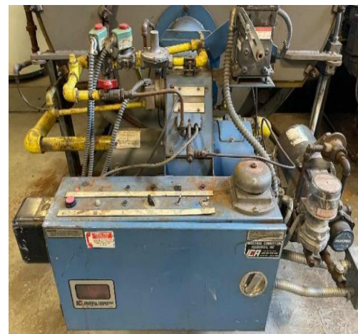
Boiler Burner Control
