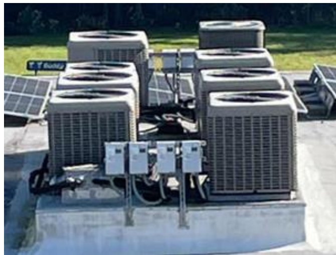
Split System AC Condensing Units
