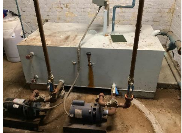
Boiler Room Condensate Pump
