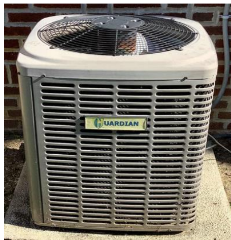
Unit Ventilator Condensing Unit
