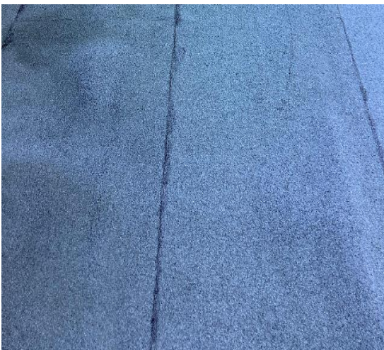
Built Up Asphalt Roof
