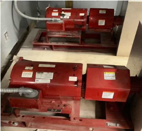
15 hp Variable Flow Condenser Water Pumps
