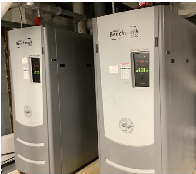
AERCO Condensing Boilers
