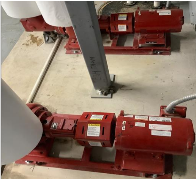
Hot Water Pumps - P5 and P6
