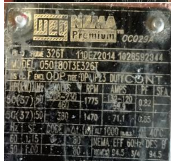
40 hp (P3 & P4) and 50 hp (P1 & P2) Variable Flow WSHP Circulation Pumps
