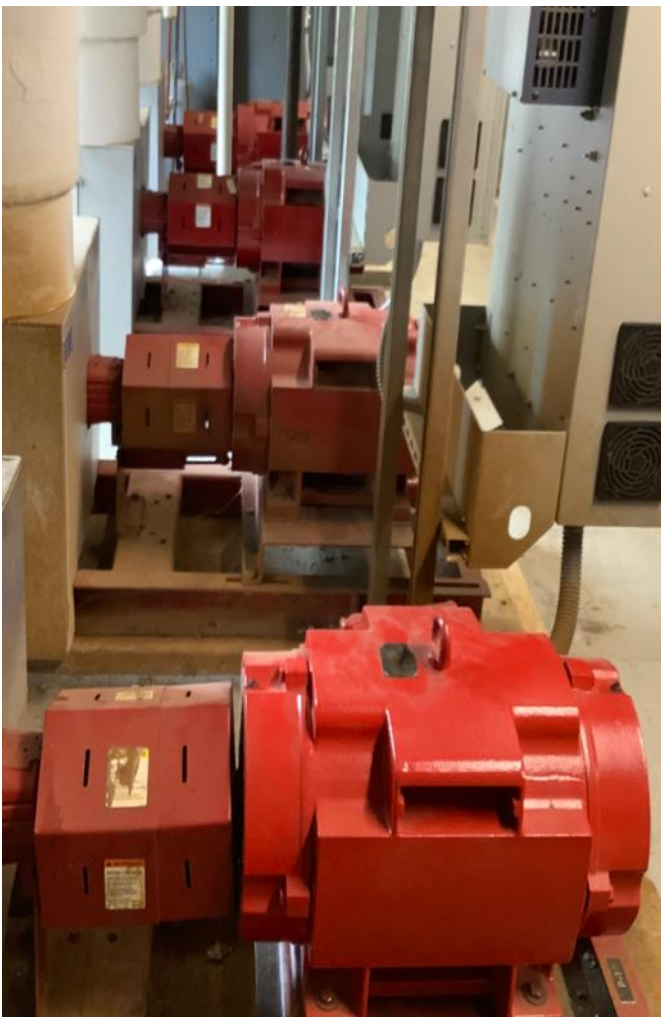
40 hp (P3 & P4) and 50 hp (P1 & P2) Variable Flow WSHP Circulation Pumps
