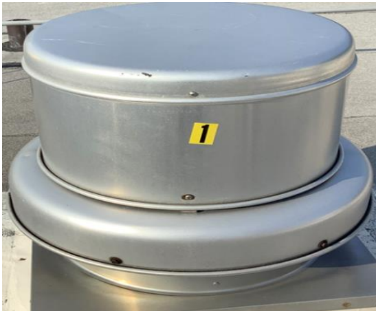
Typical Facility Exhaust Fans
