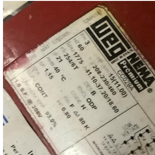
15 hp Variable Flow Condenser Water Pumps
