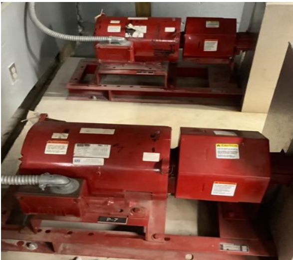
15 hp Variable Flow Condenser Water Pumps
