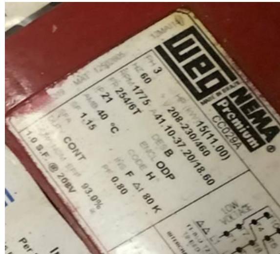
15 hp Variable Flow Condenser Water Pumps
