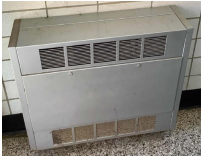
Electric Resistance Heaters
