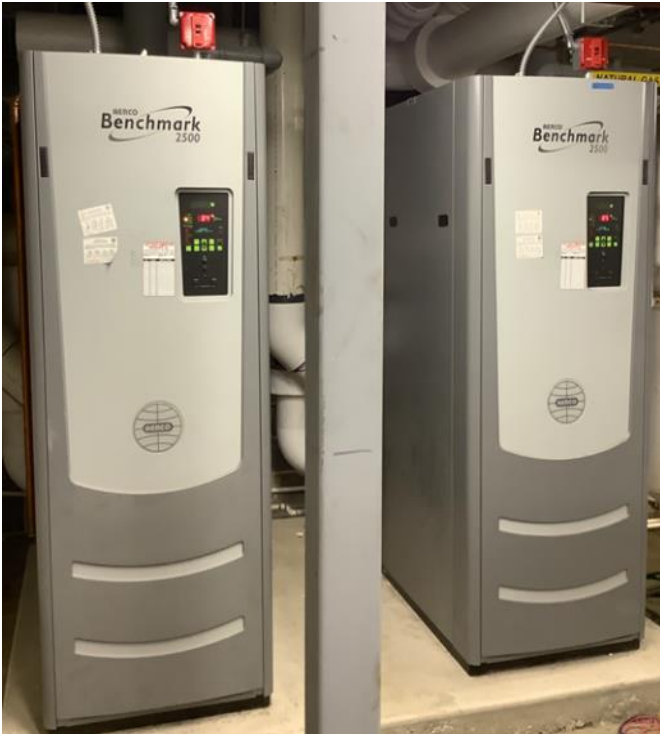
AERCO Condensing Boilers
