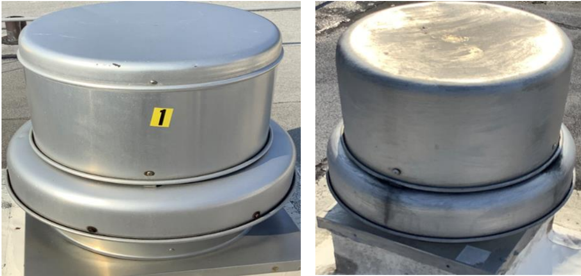
Typical Facility Exhaust Fans
