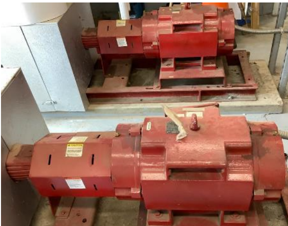
50 hp (P1 and P2) and 40 hp (P3 and P4) Variable Flow WSHP Circulation Pumps
