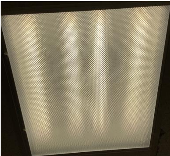
2-Foot LED Tubes Fixture
