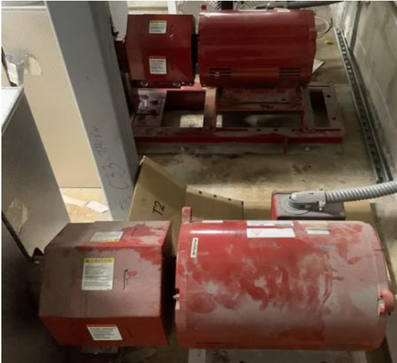
Hot Water Pumps - P5 and P6
