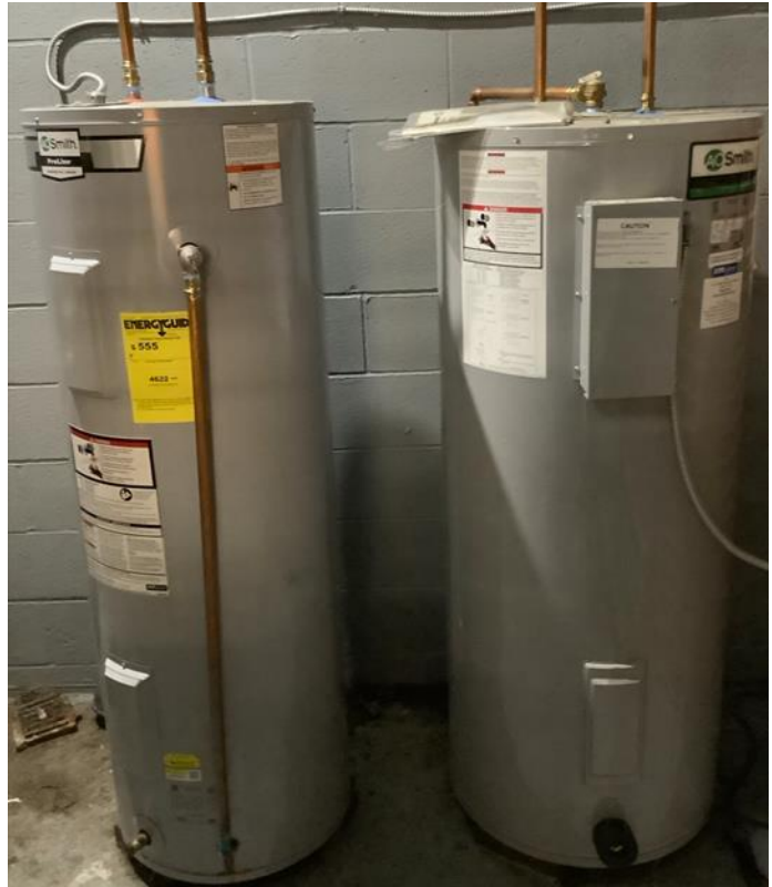
Electric Storage Tank Water Heaters
