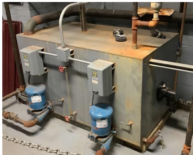
Boiler Condensate Pumps
