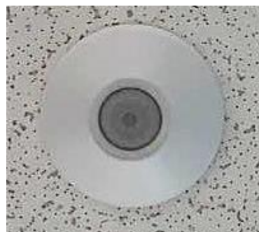
Ceiling Mounted Occupancy Sensor
