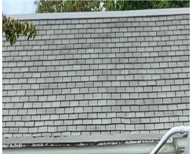
Pitched Asphalt Shingle Roof
