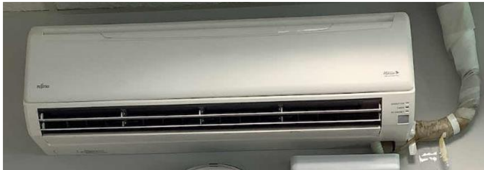
Indoor Air Source Heat Pump Unit
