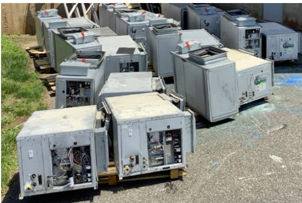
Old & Removed Tetco WSHPs
