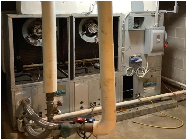
Tetco Ground Mounted WSHP
