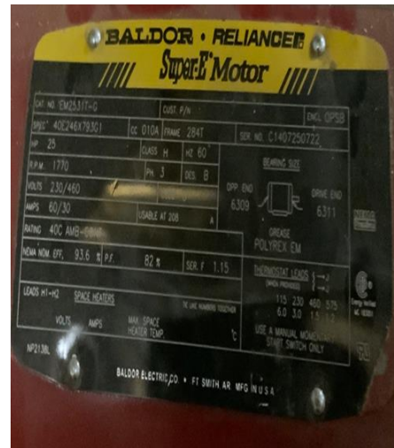
25 hp Condenser Water Pumps (P7 and P8)
