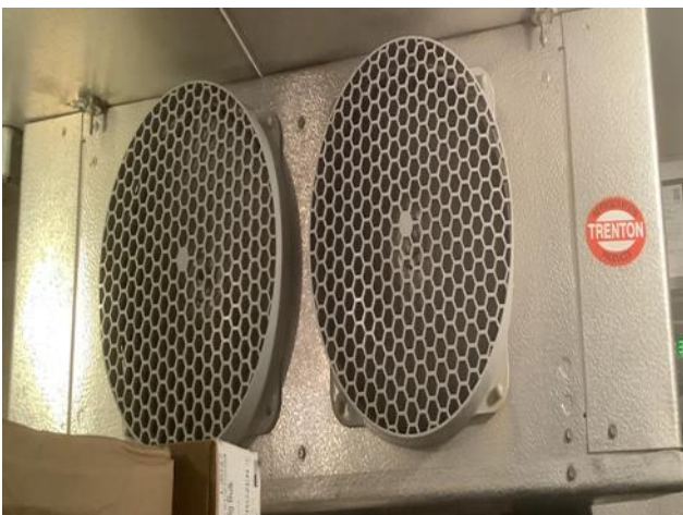
Evaporators - Medium Temperature Walk-In Freezer
