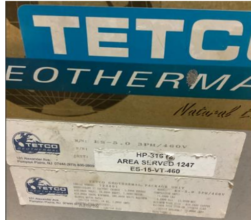
Tetco Ground Mounted WSHP
