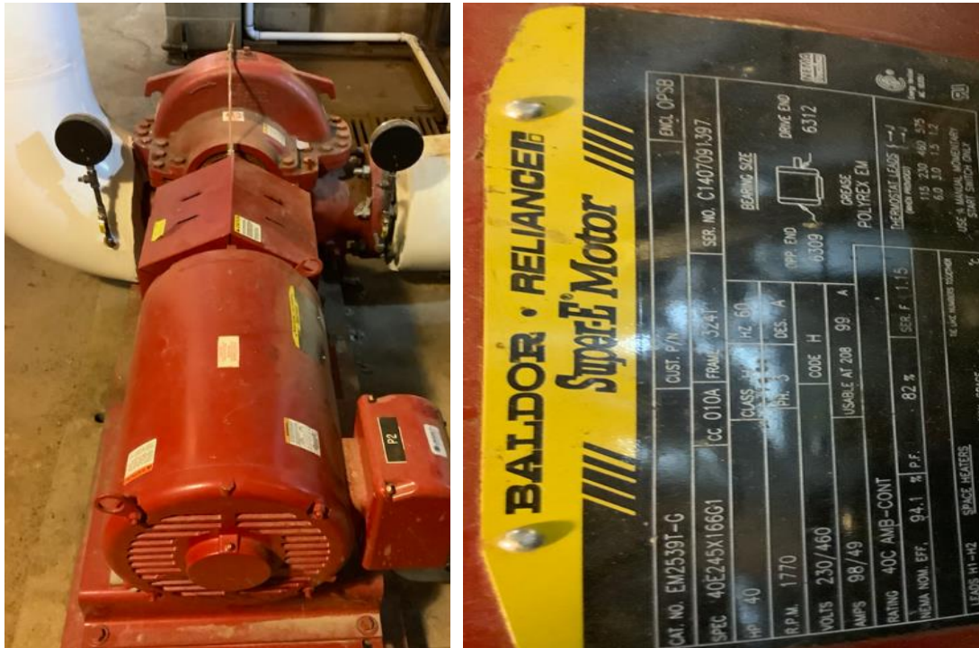
40 hp Water Circulation Pump (P2)
