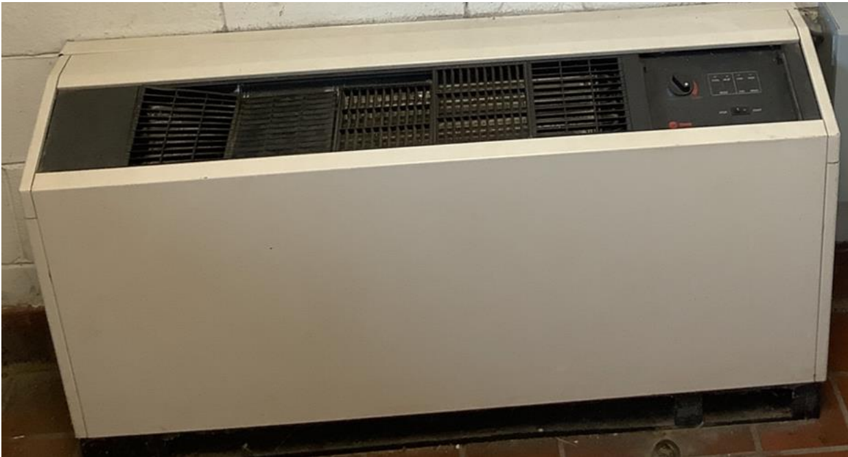
Tetco Unit Ventilator WSHP
