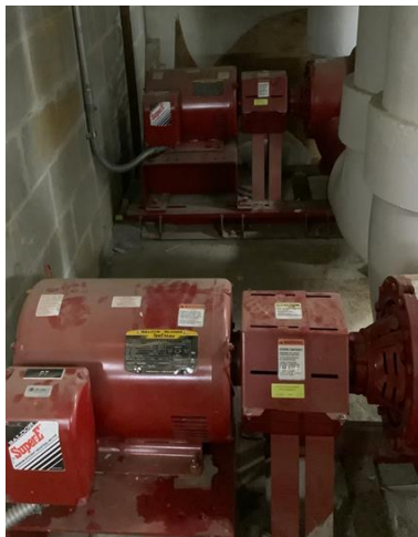
25 hp Condenser Water Pumps (P7 and P8)
