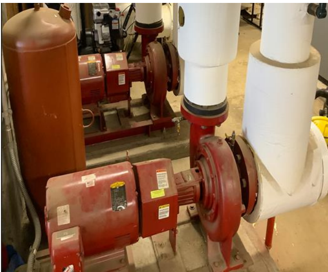
Hot Water Pumps - P5 and P6
