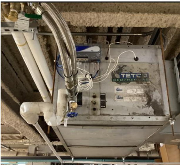
Tetco Ceiling Mounted WSHP
