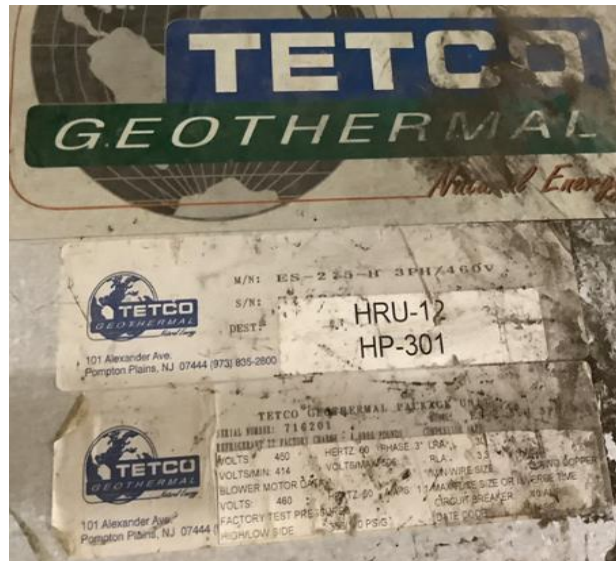
Tetco Ceiling Mounted WSHP
