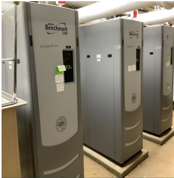
AERCO Condensing Boilers
