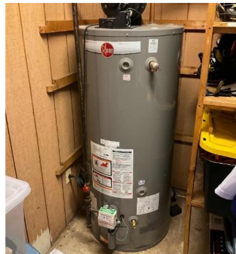
Storage tank water heater
