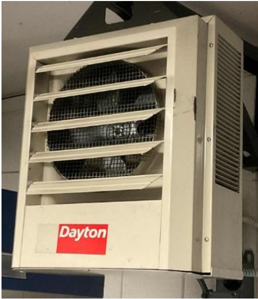
Electric resistance unit heater
