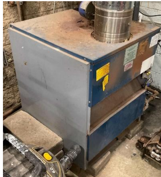
Utica Boilers hot water boiler
