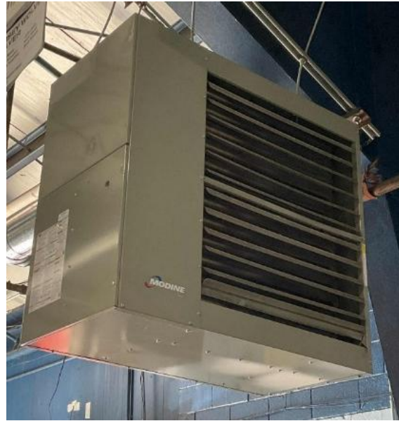
Gas powered unit heater
