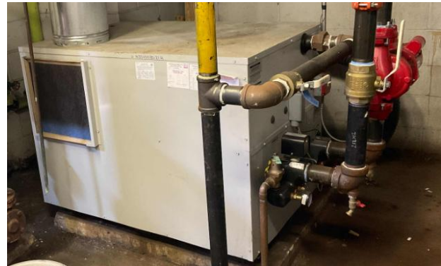
Hot Water Boilers and Heating Hot Water Pumps
