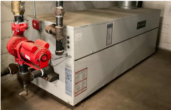
Hot Water Boilers and Heating Hot Water Pumps
