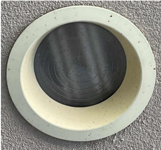
Recessed Fixture with CFLs
