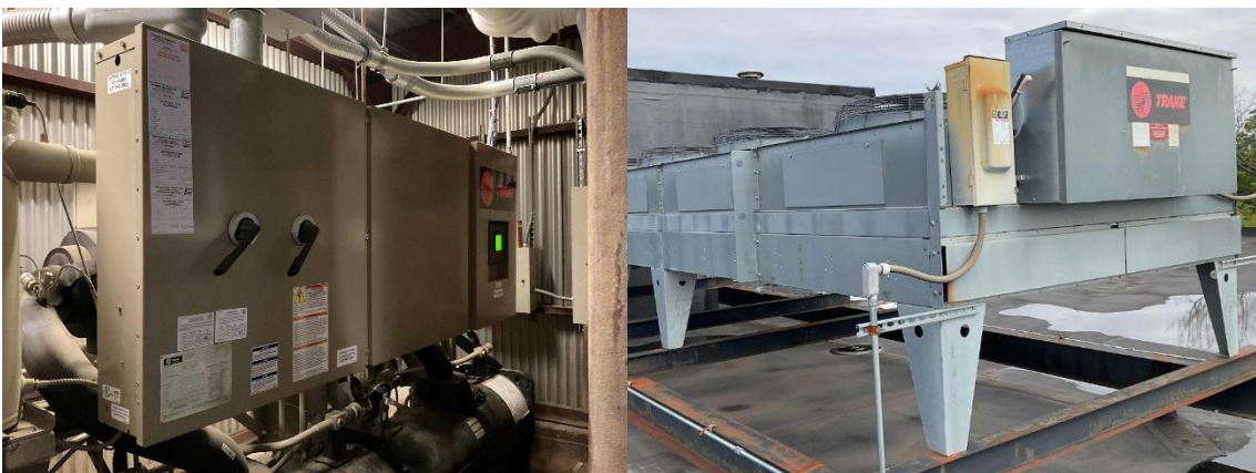
Trane air-cooled screw chiller
