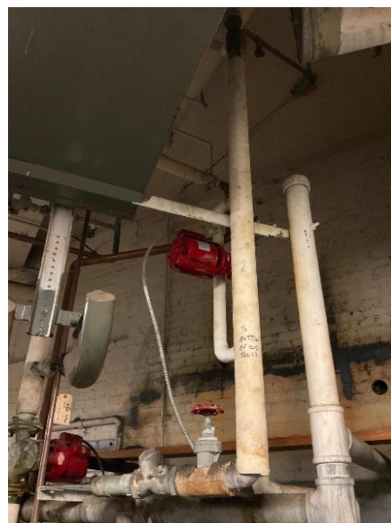
DHW Circulating Pumps
