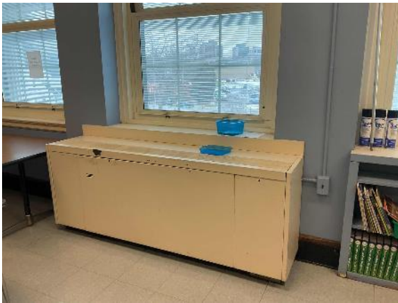
Typical Classroom Unit Ventilator
