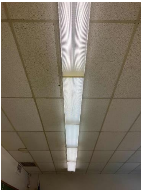
Linear Fluorescent T8 Lamps
