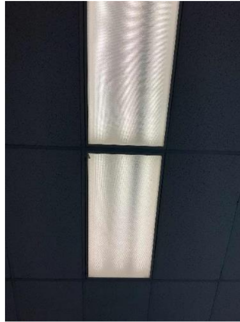
Linear Fluorescent T8 Lamps
