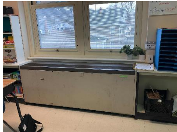
Typical Classroom Unit Ventilator
