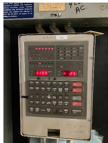
Boiler Control System
