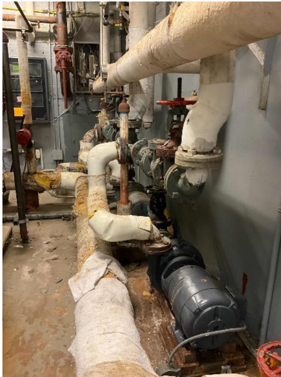
Boiler HW Pumps
