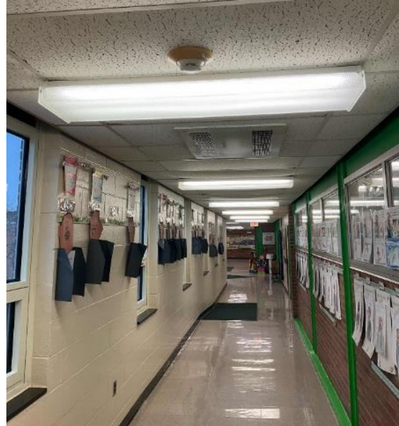
Corridor- Linear Fluorescent Fixtures
