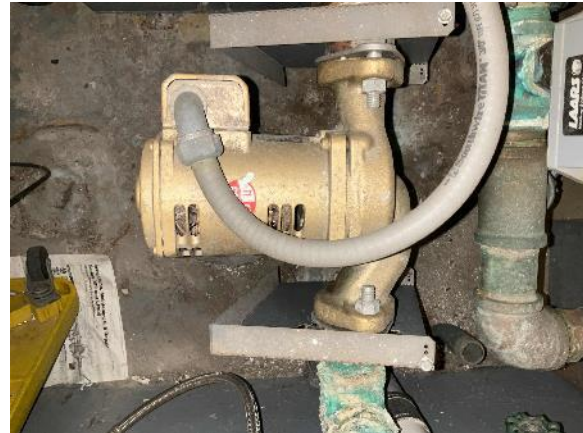
DHW Circulation Booster Pump
