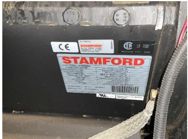
Emergency Generator-Nameplate
