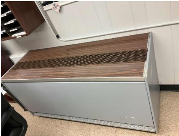
Typical Classroom Unit Ventilator
