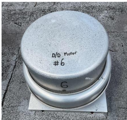
Typical Exhaust Fan
