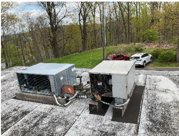
Outdoor Condensing Unit- Walk-In Cooler and Freezer
