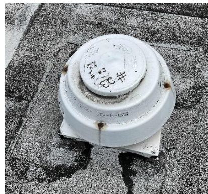
Typical Exhaust Fan
