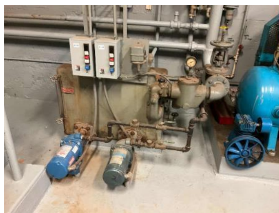
Boiler Condensate Return System-LLC
