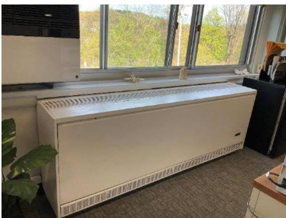
Typical Unit Ventilator-LLC
