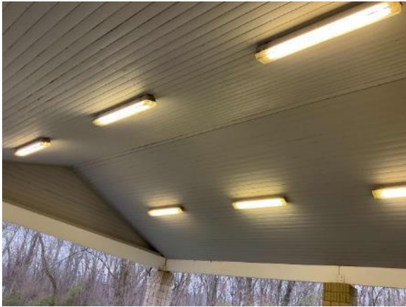
T8 Fluorescent Lamps Exterior Canopy- Harter Road
