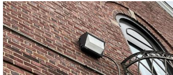
Exterior LED Wall Pack Fixtures-LLC
