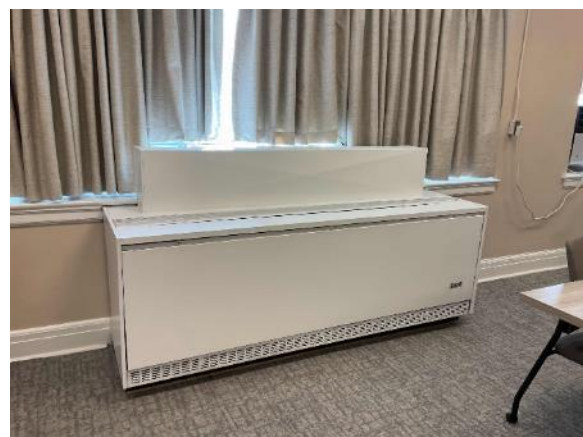
Typical Unit Ventilator-LLC
