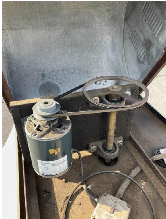
Typical Exhaust Fan Motor-LLC
