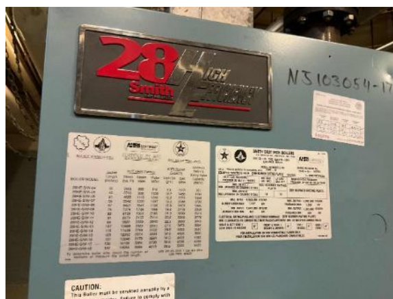
Steam Boiler Nameplate-LLC
