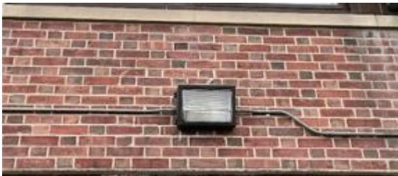
Exterior HID Wall Pack Fixtures-LLC
