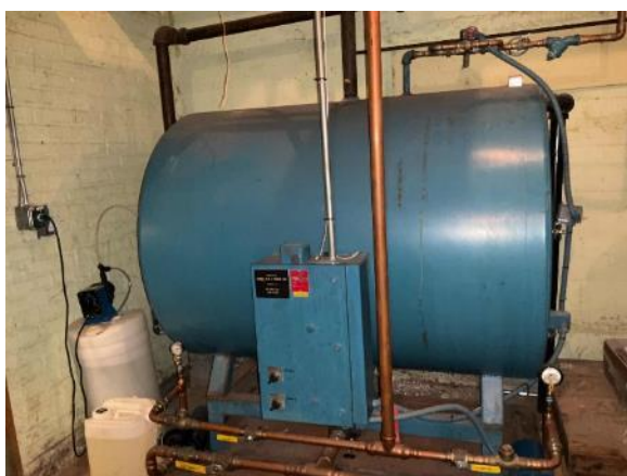
Boiler Feed Water System-LLC
