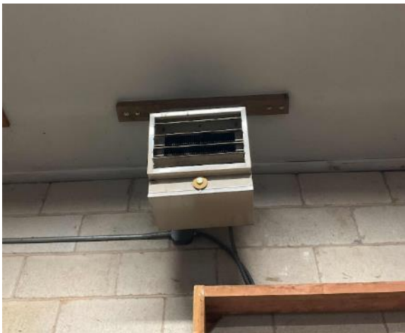
Harter Road Main Garage – Unit Heater
