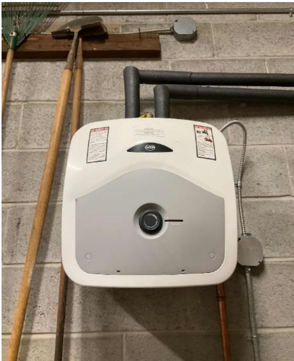
Domestic Hot Water Heater - Harter Road
