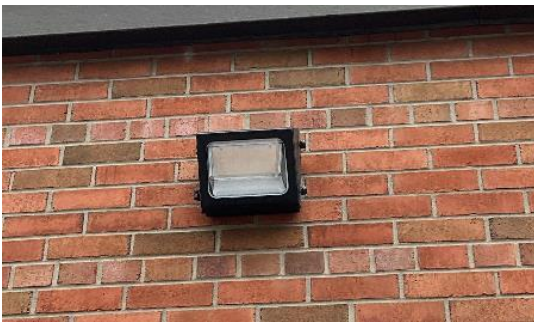
Exterior LED Wall Pack Fixture
