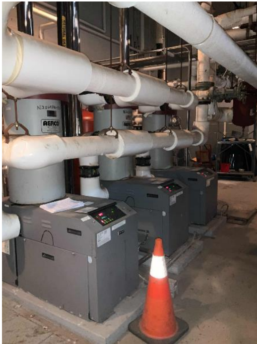
Hydronic Boiler- Aerco
