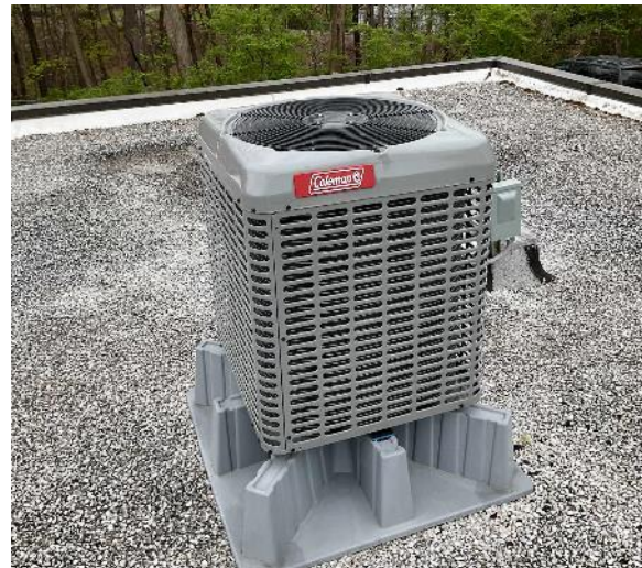
Outdoor Condensing Unit- Band Room
