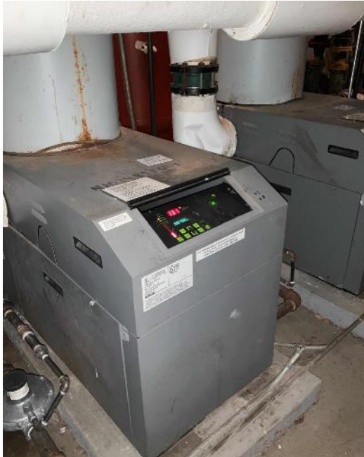
Hydronic Boiler- Aerco
