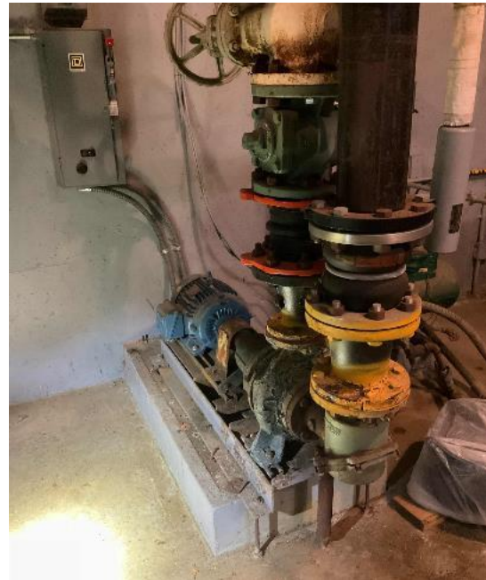
Boiler Hot Water Pump
