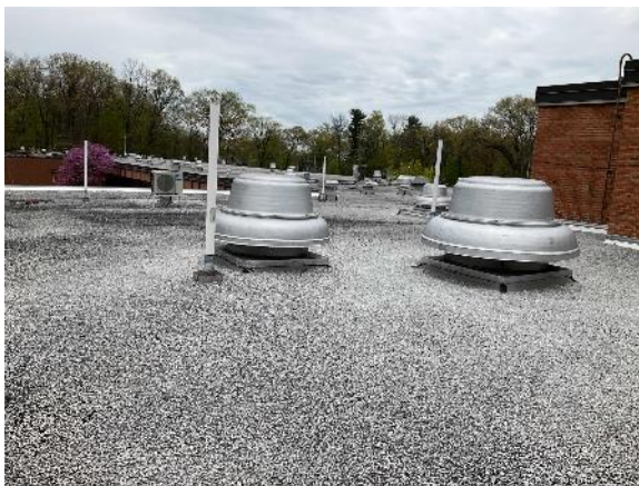
Typical Rooftop Exhaust Fan
