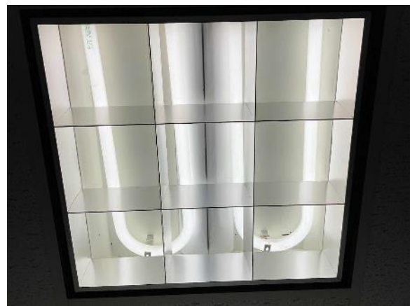
Typical T8 U-bend Fluorescent Fixture
