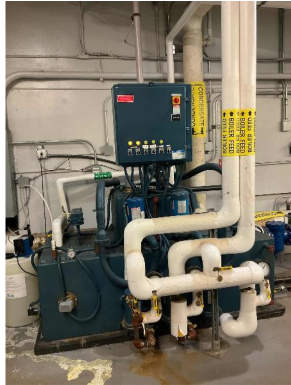
Feed Water and Condensate Return Loop
