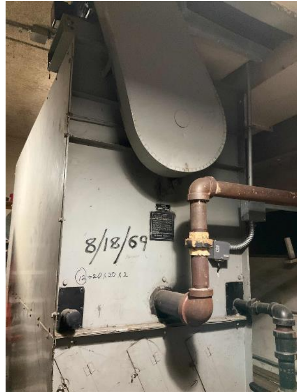
Air Handling Unit - Storage Room
