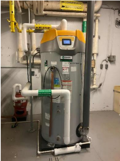
Gas Fired Storage Tank Heater
