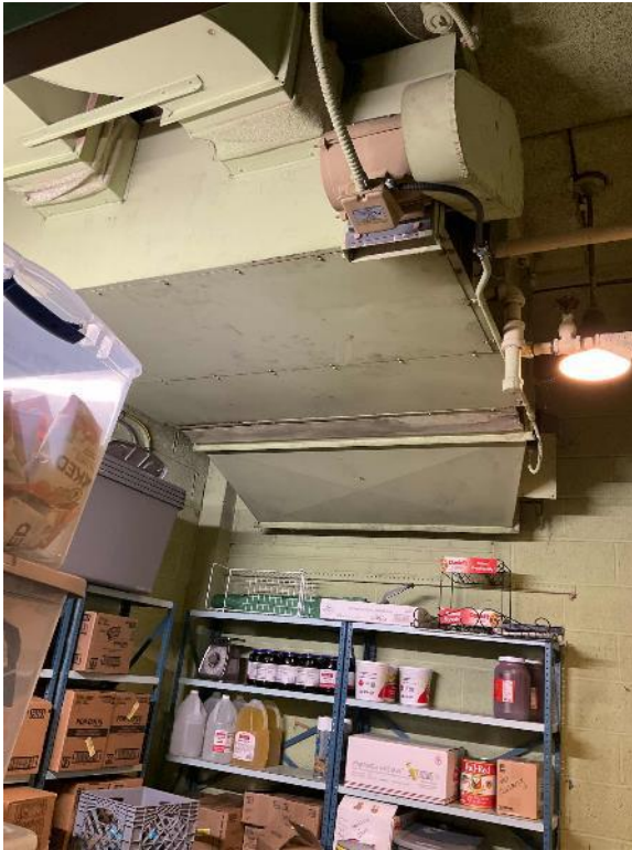
Air Handling Unit - Kitchen Area
