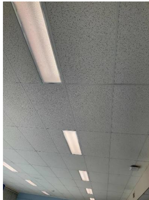
LED Linear Tube Fixture
