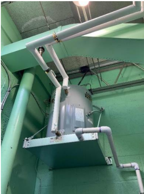
Electric Storage Water Tank Heater
