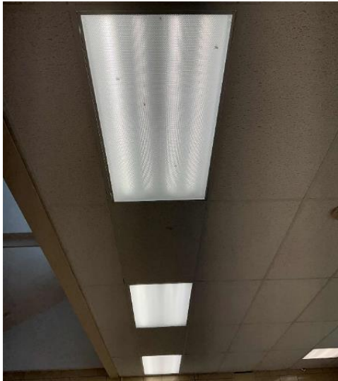
Typical LED Linear tube Fixtures
