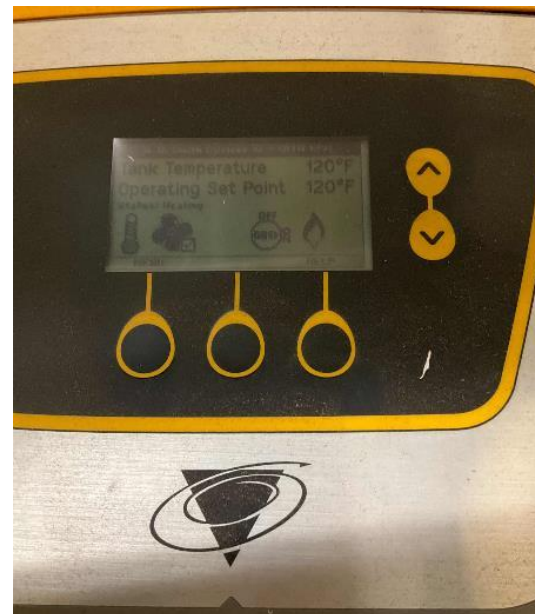
Domestic Hot Water Heater- Setpoint
