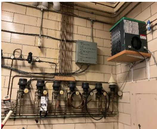
Pneumatic System with Refrigerant Dryer
