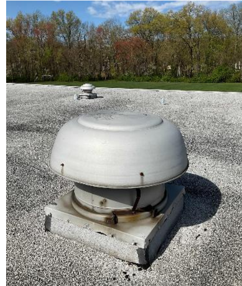
Typical Rooftop Exhaust Fans
