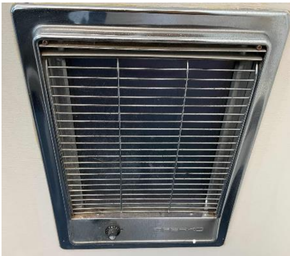
Electric Resistance Heater
