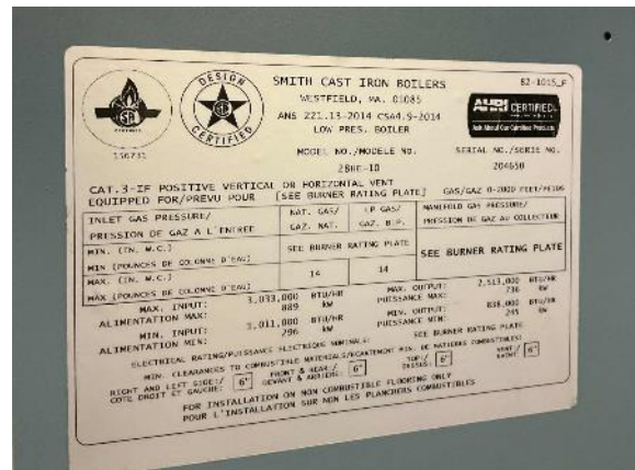
Boiler Nameplate-Boiler 1
