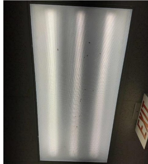
Typical LED Linear tube Fixtures
