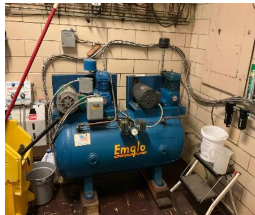
Air Compressor- Pneumatic System
