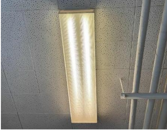
Typical T8 Fluorescent Fixture
