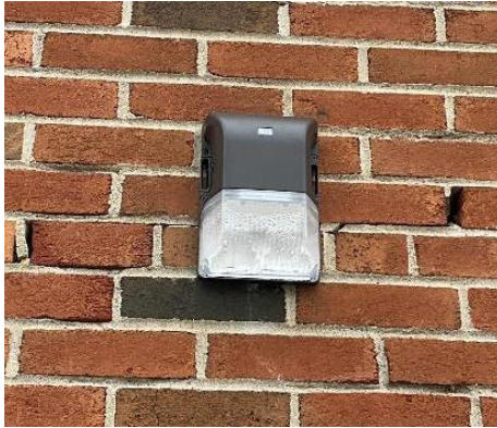
Exterior LED Wall Packs
