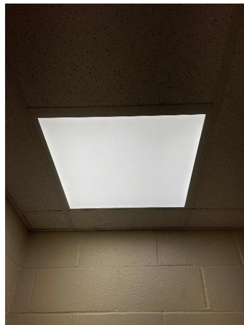
LED 2-foot x 2-foot Fixture
