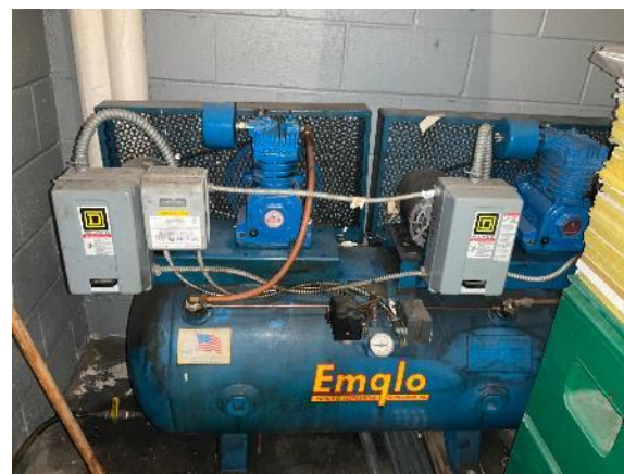
Air Compressor- Pneumatic System
