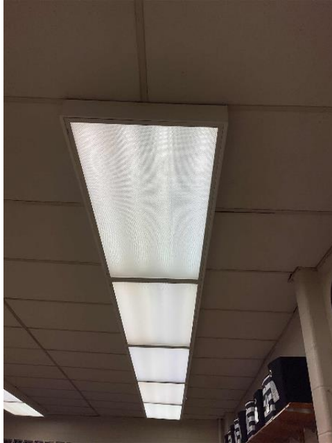
Linear Fluorescent T8 Lamps
