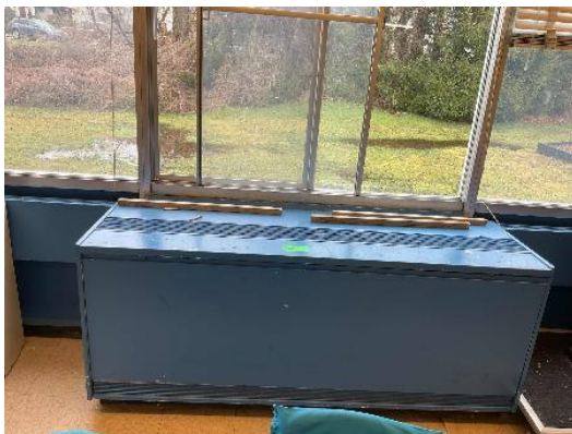
Typical Unit Ventilator
