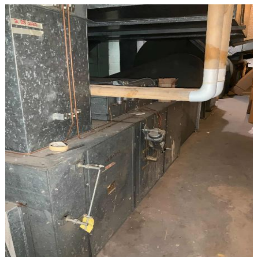
Air Handling Units-Attic Area
