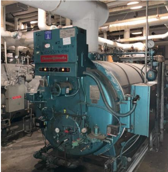
Hydronic Boiler- Cleaver Brooks-CB 200-100
