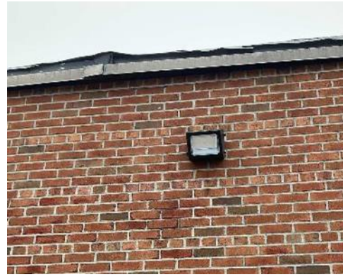
Exterior LED Wall Packs
