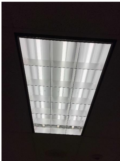
Linear Fluorescent T8 Lamps
