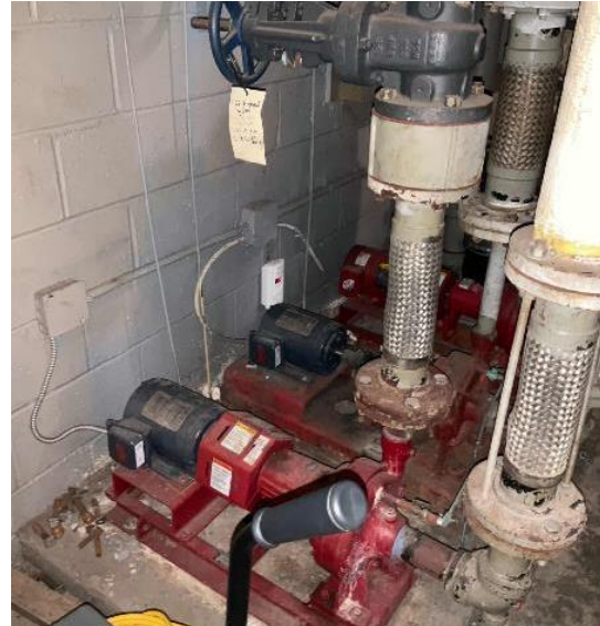
Boiler Hot Water Pump
