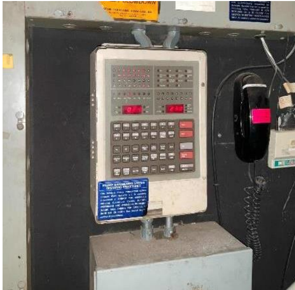
Boiler Control System
