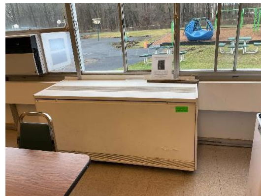
Typical Unit Ventilator
