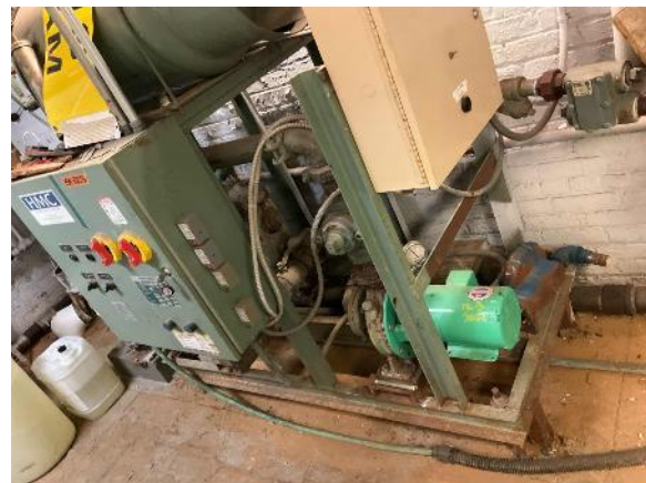
Heat Exchanger- Steam to Hot Water
