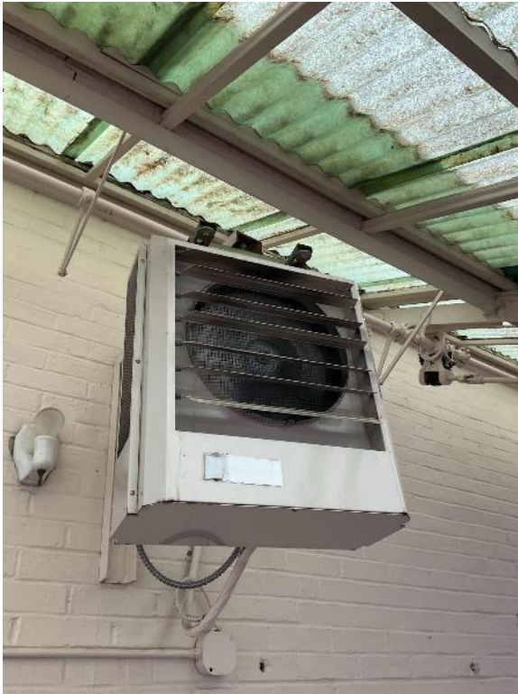
Electric Resistance Heater
