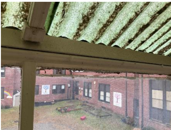
Green House Envelope with Infiltration Gap
