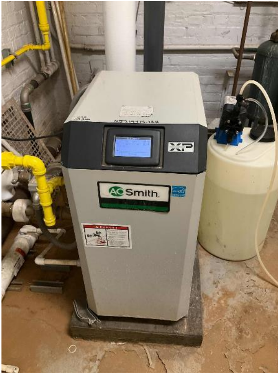
Gas Fired Hot Water Heater
