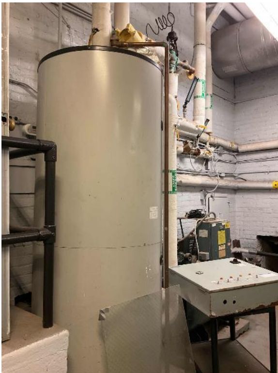
Storage Tank Heater
