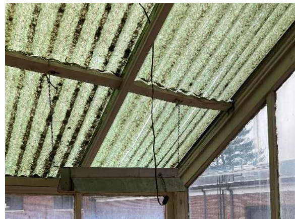
Green House Envelope with Infiltration Gap
