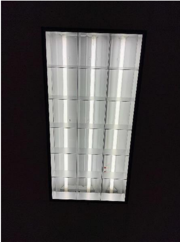
Linear T8 Fluorescent Fixtures
