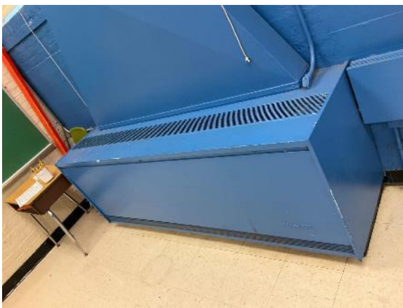
Typical Unit Ventilator
