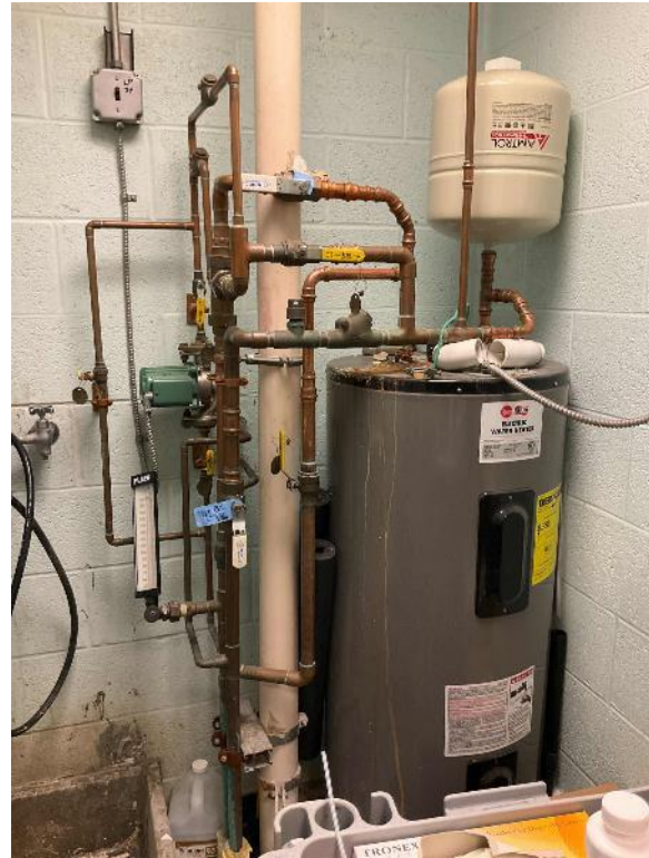
Electric Storage Tank Heater
