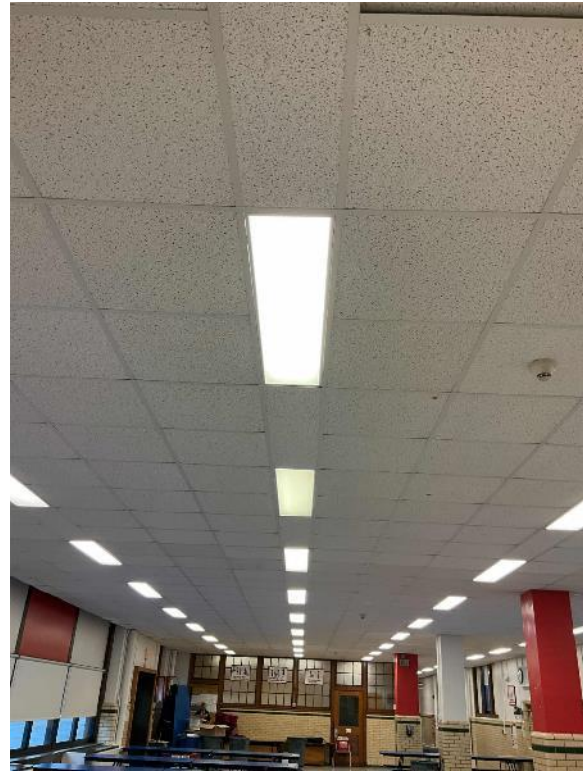
Linear T8 Fluorescent Fixtures
