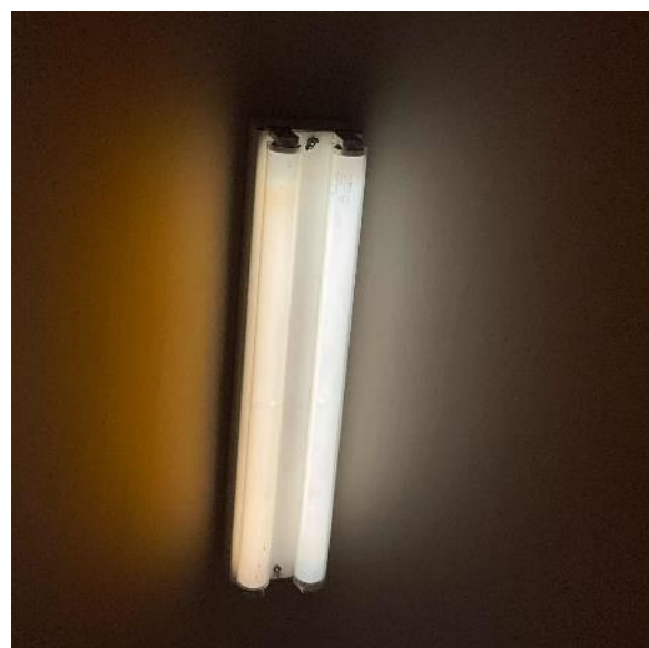
Linear T12 Fluorescent Fixtures
