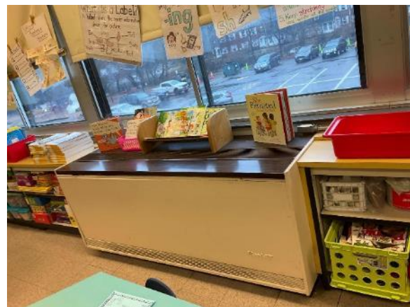
Typical Unit Ventilator
