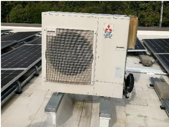
Mini-Split Air Conditioning Unit
