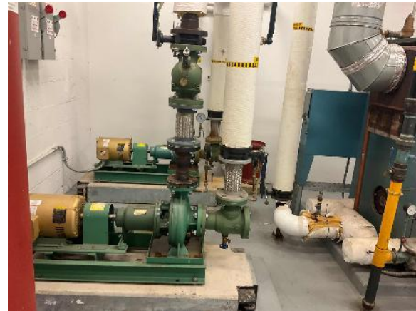
Hot Water Heating Pump
