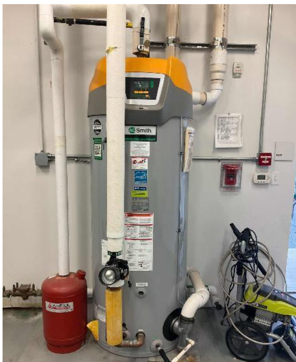
Gas-fired Storage Water Tank Heater
