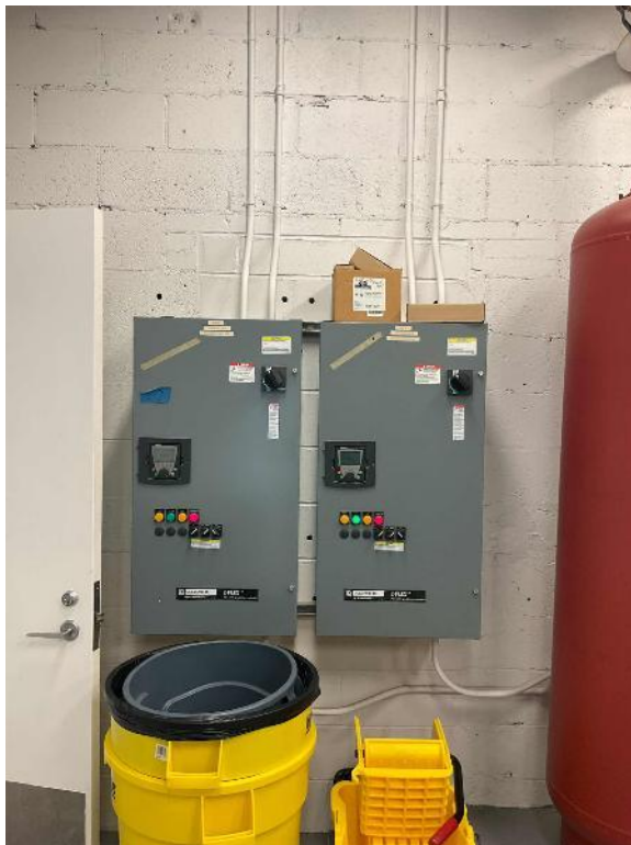
Hot Water Heating Pump: VFD
