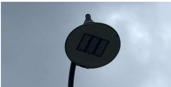
Exterior Pole Mounted LED Fixtures
