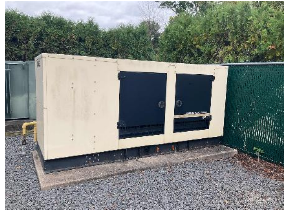
Natural Gas-fired Emergency Generator
