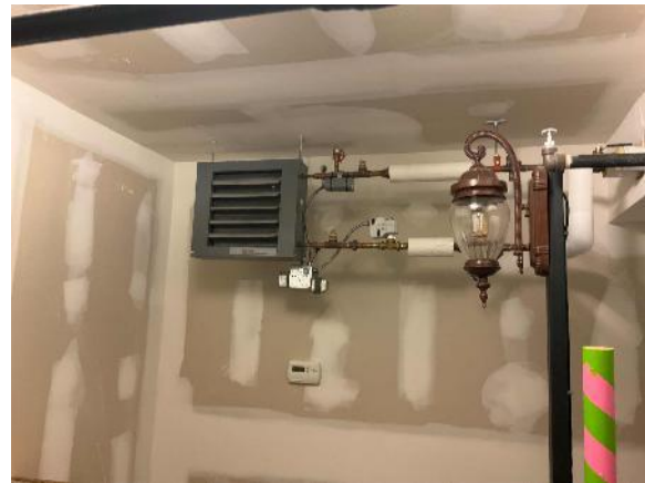
Unit Heater: Hot Water
