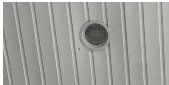
Exterior CFL Can Fixture
