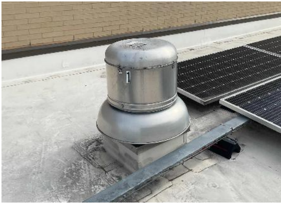
Typical Exhaust Fan
