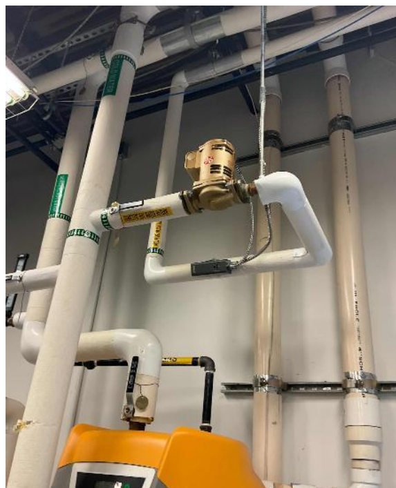
DHW Recirculation Pump
