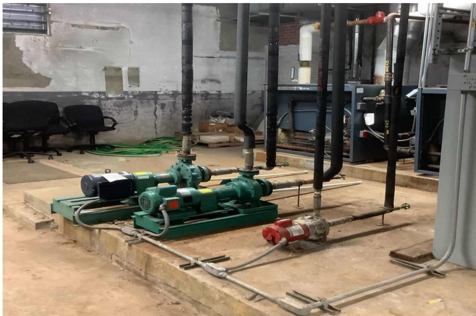
Heating Hot Water Pumps
