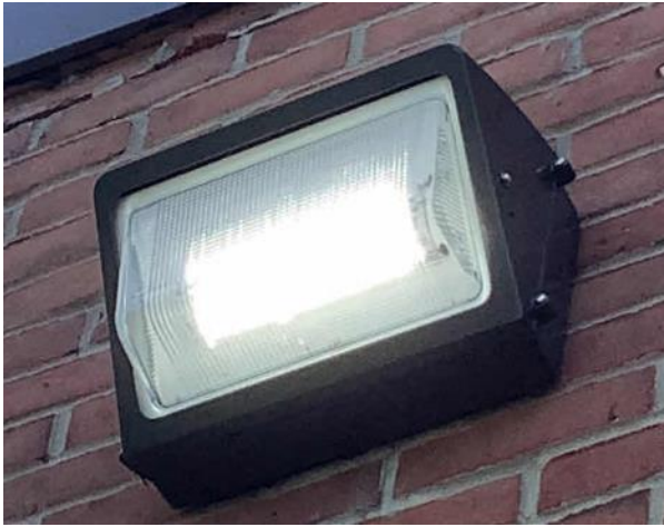
Exterior LED Fixture
