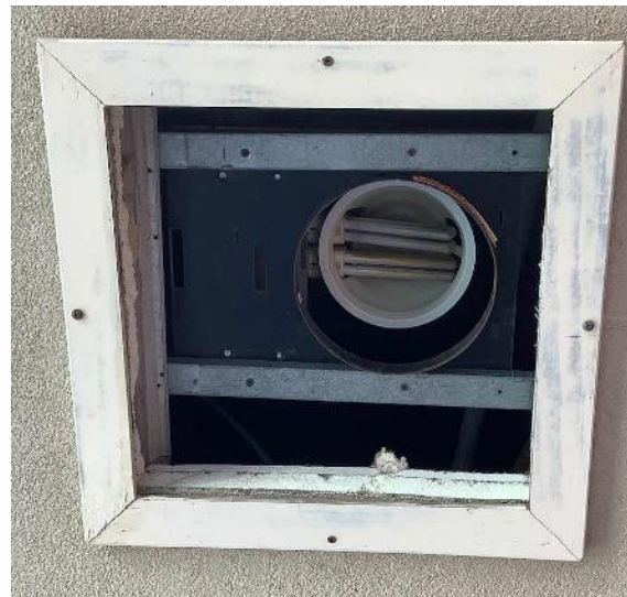
Exterior CFL Fixtures
