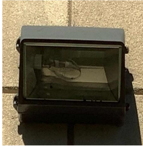
Exterior MH Fixture
