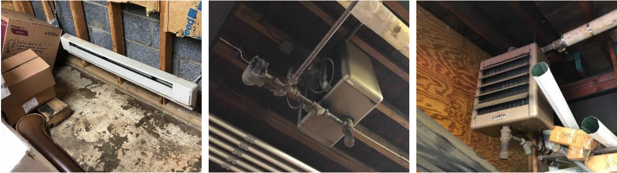
Warehouse Electric Resistance Heater and Unit Heaters
