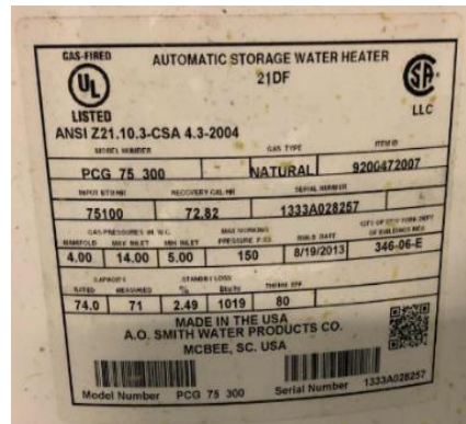
Field House Gas-fired Storage Water Heater
