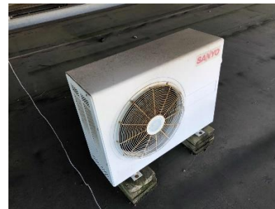
Field House Outdoor Condensing Unit
