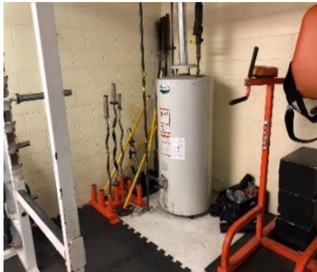
Field House Gas-fired Storage Water Heater
