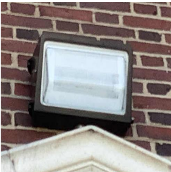
Exterior LED & MH Fixtures
