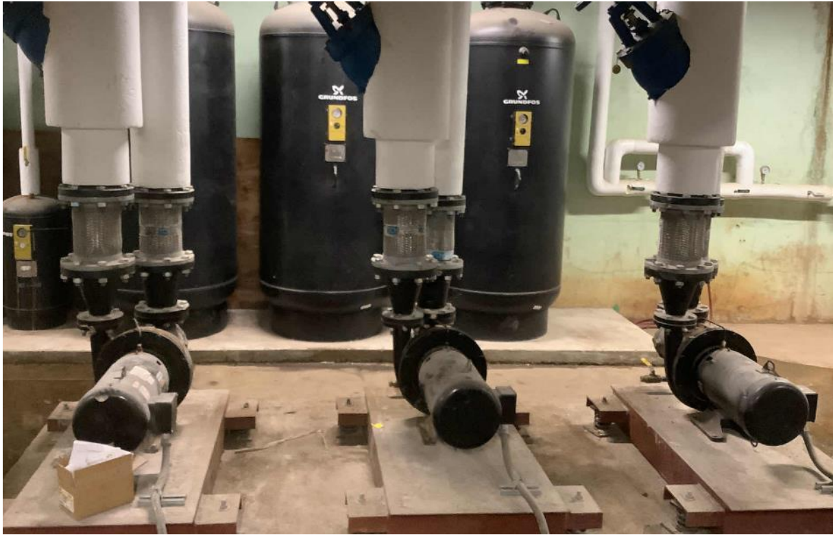
Heating Hot Water Pumps
