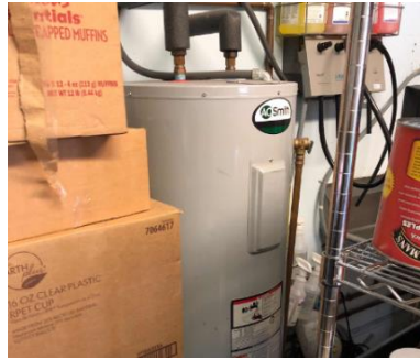
Storage Tank Water Heaters
