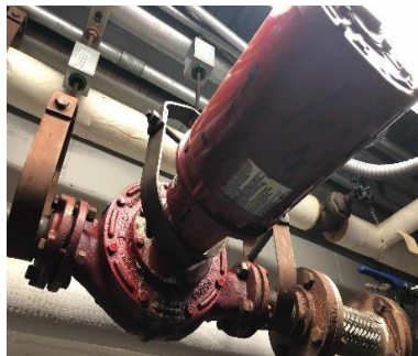
Heating Hot Water Pumps
