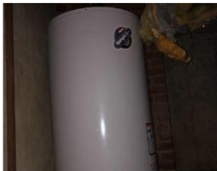
Storage Tank Water Heater
