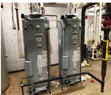
Storage Tank Water Heaters
