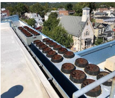
Air-Cooled Screw Chillers
