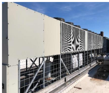
Air-Cooled Screw Chillers
