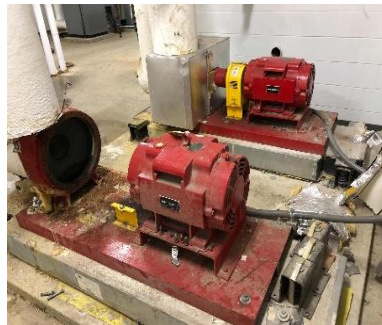
Heating Hot Water Pumps for Addition
