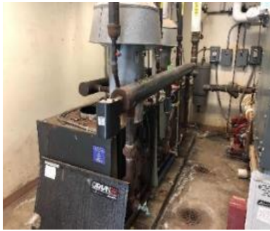
Hot Water Boiler
