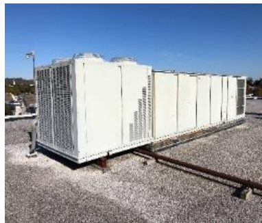
Roof Top Packaged Units
