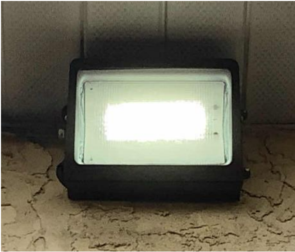
Exterior LED Fixture
