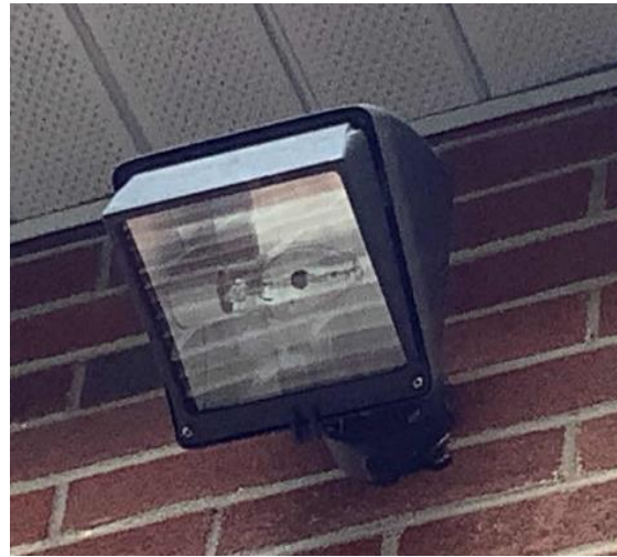
Exterior MH Fixture
