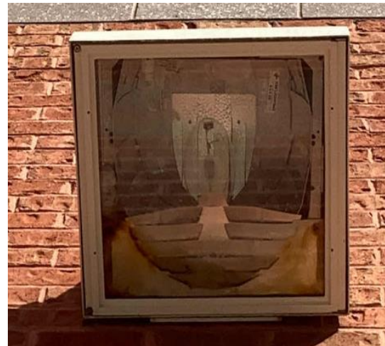
Exterior MH Fixture
