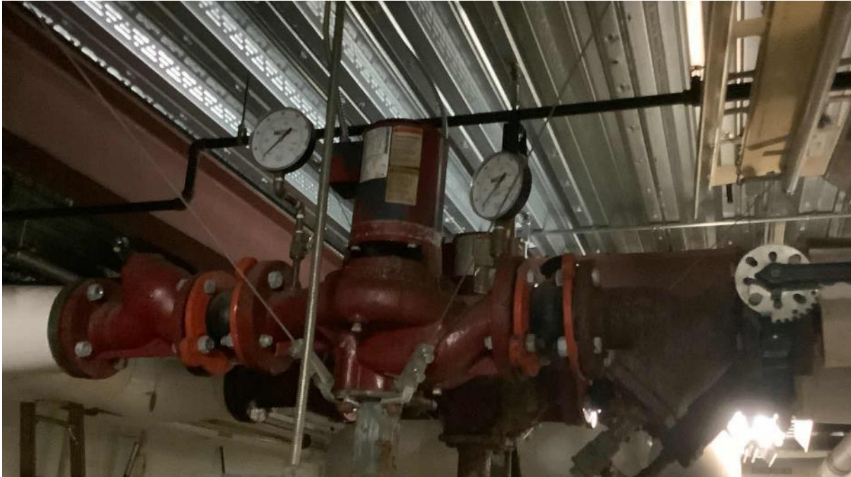
Heating Hot Water Pumps
