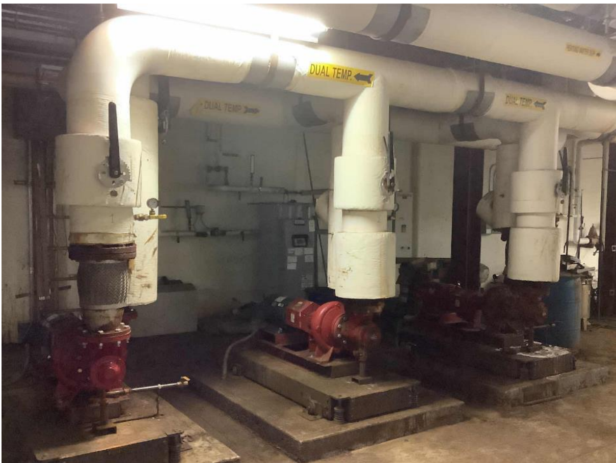
Dual Temperature Pumps
