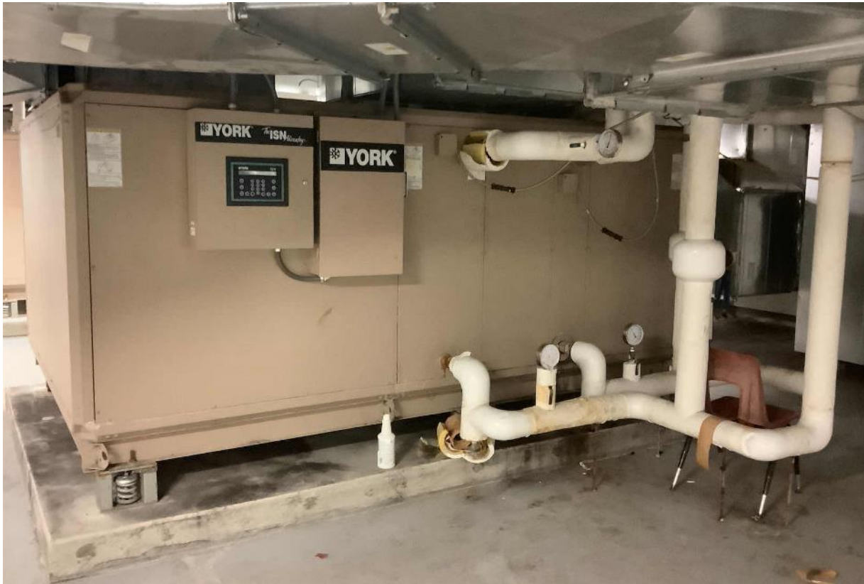
Air Handling Unit (AHU-3)
