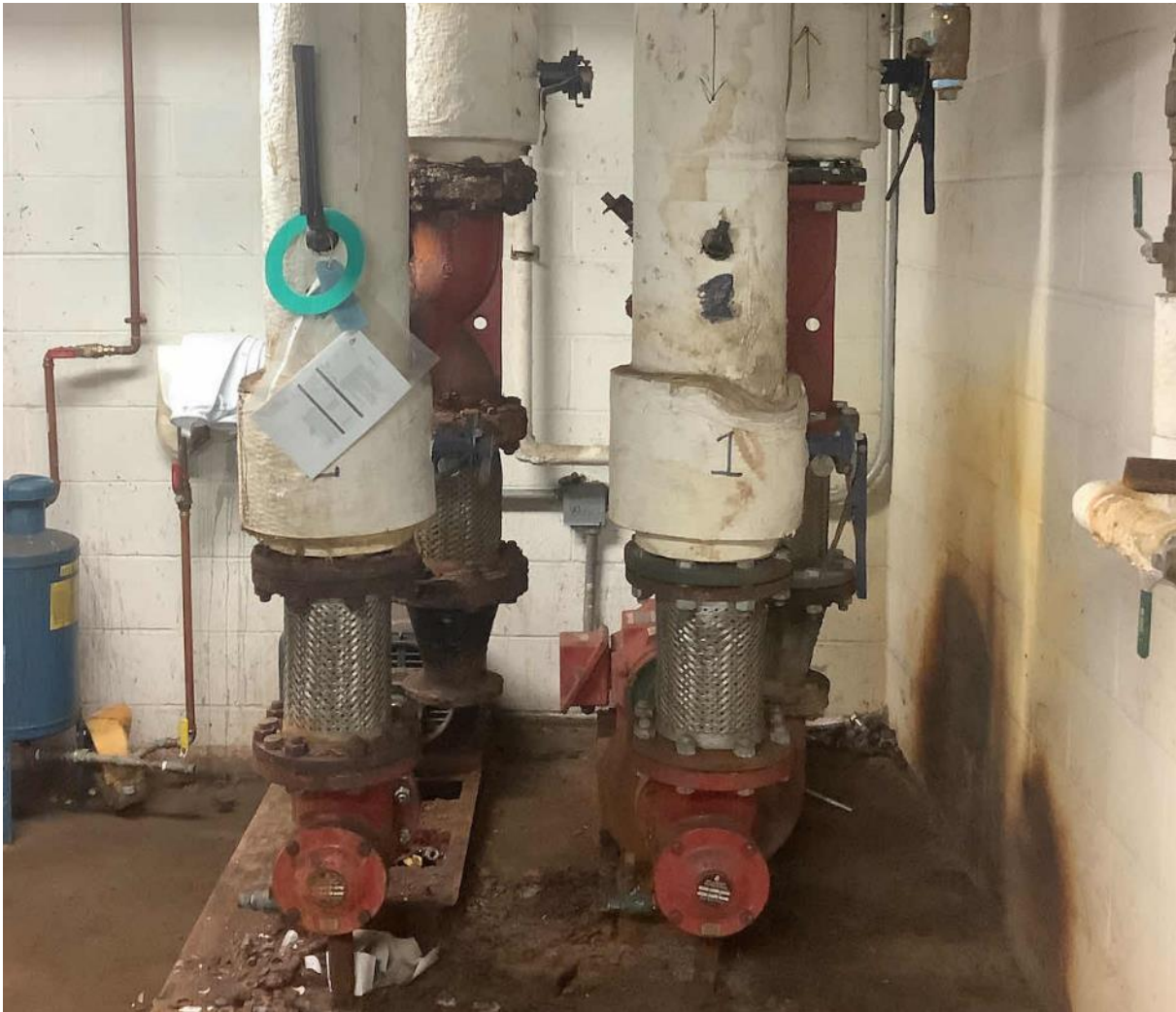
Heating Hot Water Pumps
