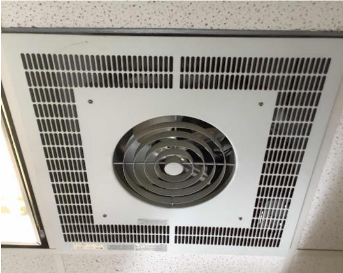
Electric Resistance Heaters
