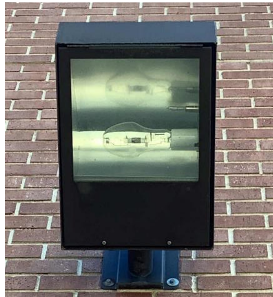
Exterior MH Fixture
