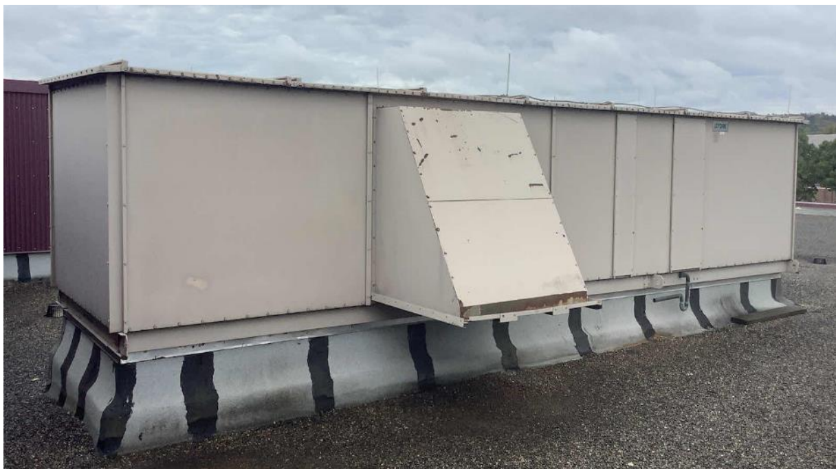
Air Handling Unit (AHU-4)
