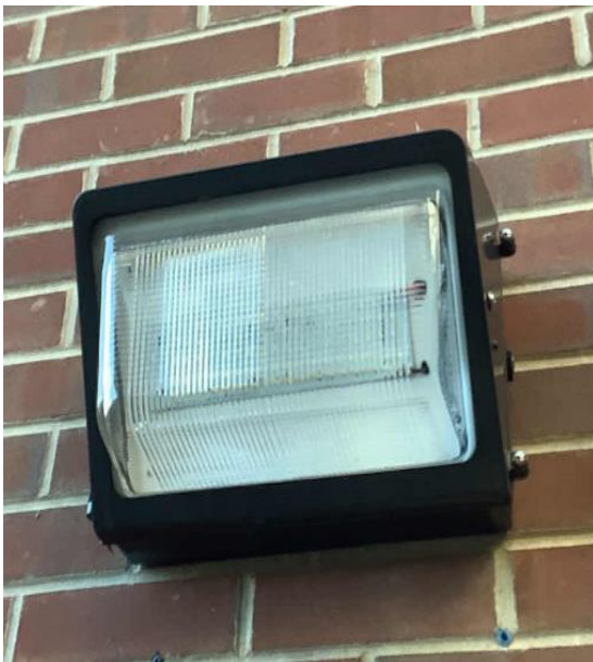
Exterior LED Fixture
