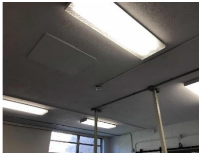
Surface Mounted Fixtures
