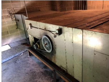
Air Handling Unit (AHU)
