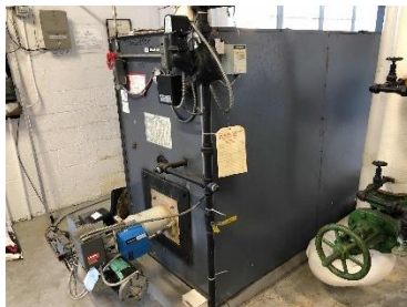
Hot Water Boiler
