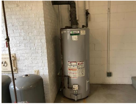
Storage Tank Water Heater
