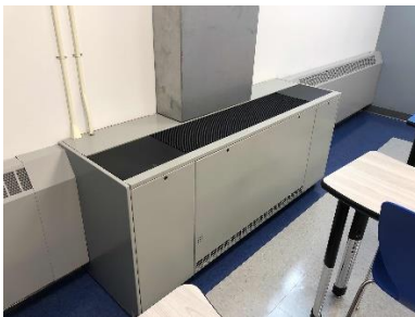
New Unit Ventilator
