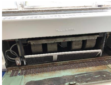
Typical Unit Ventilator
