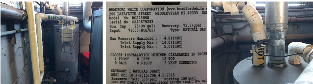
DHW unit, unit label, and pipe wrap
