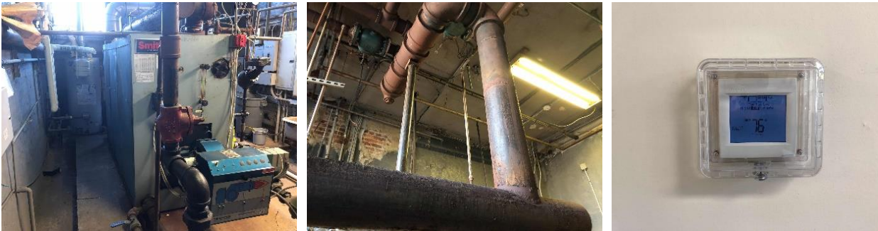
Boiler, unwrapped steam pipes, and digital thermostat
