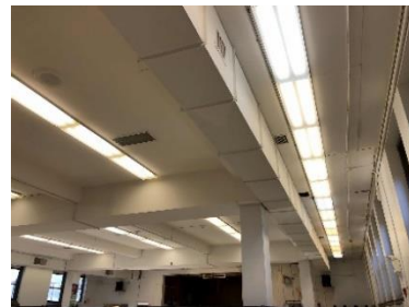
Linear fluorescent surface mounted and recessed fixtures
