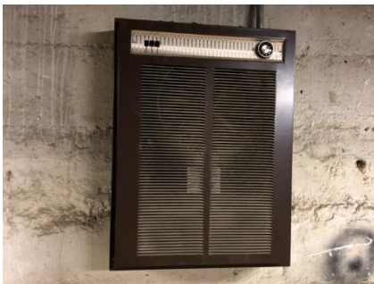
Electric Resistance Heaters
