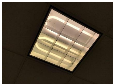
Recessed U-bend Fluorescent Fixture
