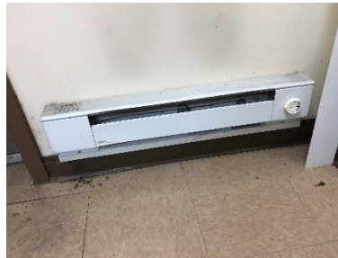
Electric Baseboard Heating
