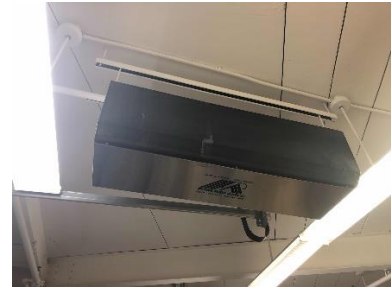
Hanging Electric Unit Heater
