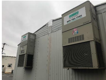
Packaged Units on Detached Trailer
