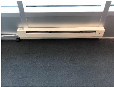
Electric Baseboard Heating
