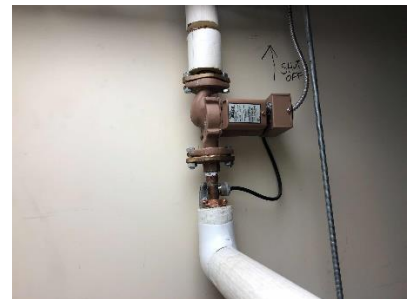
Domestic Hot Water Circulation Pump
