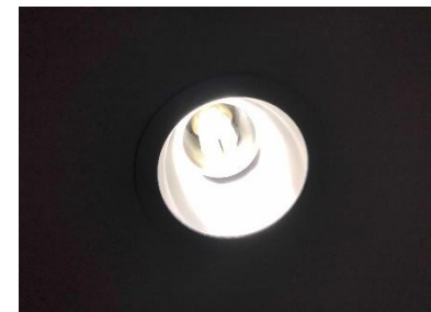
Recessed Can Fixture
