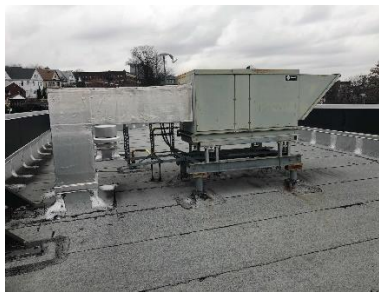
Gas-fired Makeup Air Units
