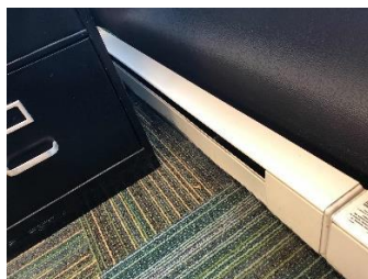
Electric Resistance Baseboard Heat
