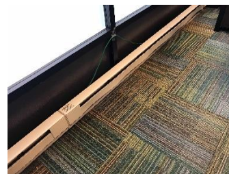
Electric Resistance Baseboard Heat
