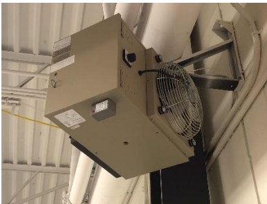
Electric Resistance Heating Units in Mechanical Space and Corridor, and Suspended Gas-fired Furnace
