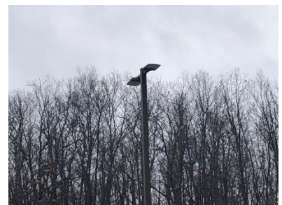
Pole Lights Retrofitted with LED Lamps and LED Pole Light Fixture
