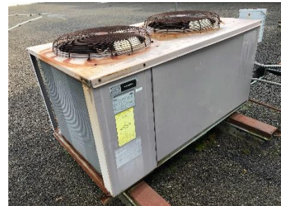
Remote Outdoor Condensing Unit
