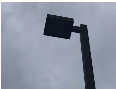
Pole Lights Retrofitted with LED Lamps and LED Pole Light Fixture
