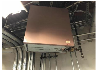
Electric Resistance Heating Units in Mechanical Space and Corridor, and Suspended Gas-fired Furnace
