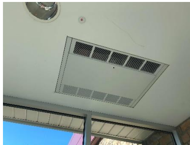
Electric Resistance Heating Units in Mechanical Space and Corridor, and Suspended Gas-fired Furnace
