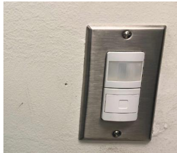
Wall Switch Occupancy Sensor
