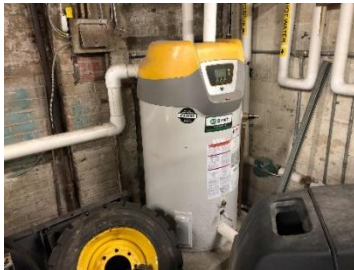
Gas-fired Storage Water Heater
