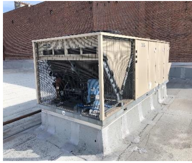
Packaged Roof Top Units
