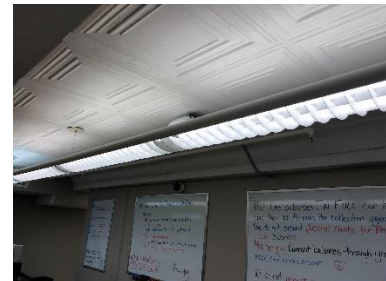
Linear Fluorescent Parabolic Fixtures Pendent and Recessed Mounted
