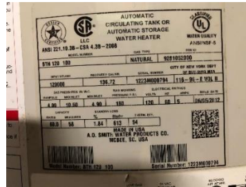
Gas-fired Storage Water Heater
