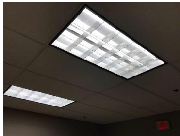
Linear Fluorescent Parabolic Fixtures Pendent and Recessed Mounted
