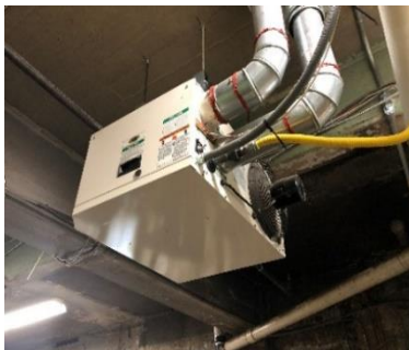
Suspended Gas-fired Furnace
