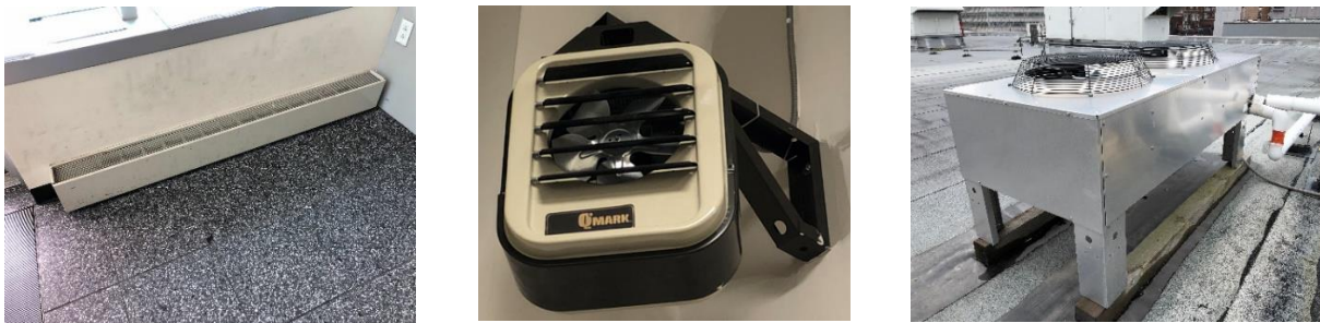
Electric Resistance Heaters
