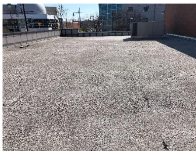
Flat roof covered with rolled asphalt
