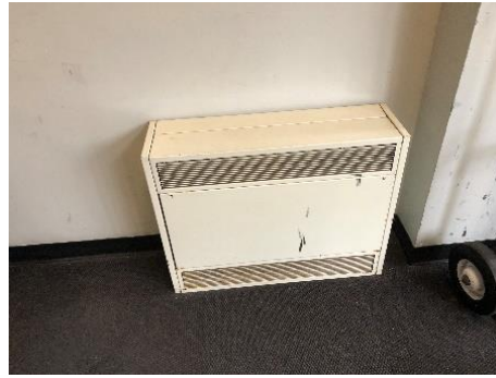
Electric Resistance Fan Coil Unit
