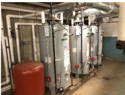
Gas-Fired Storage Water Heaters
