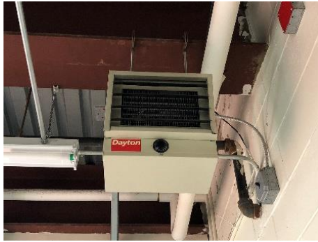
Electric Resistance Unit Heater
