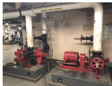
Heating Hot Water Pump
