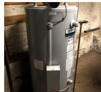
Gas-Fired Storage Water Heater
