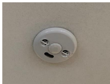
Ceiling Mounted Occupancy Sensor
