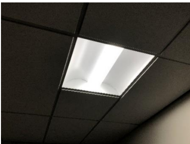
2-foot x 2-foot LED Fixture
