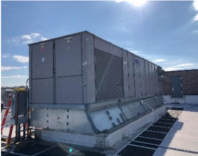
Packaged Roof Top Unit (RTU)
