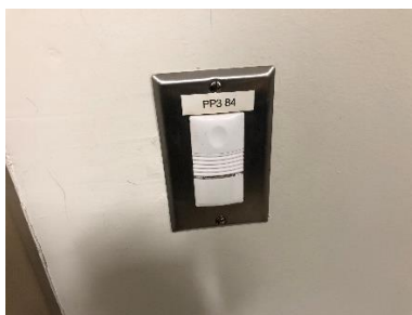
Wall Mounted Occupancy Sensor
