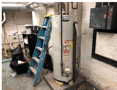
Gas-fired Storage Water Heater
