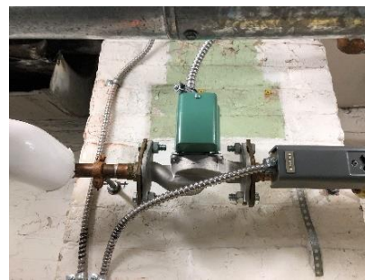
Domestic Hot Water Circulation Pump
