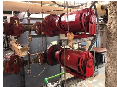
Heating Hot Water Pumps
