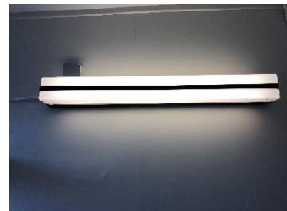
Linear Fluorescent Surface Mounted Fixture
