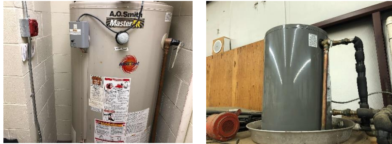
Storage Tank Water Heaters
