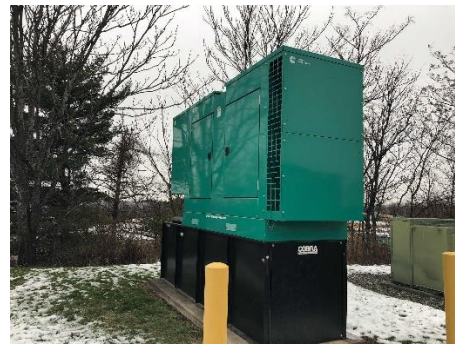
Ground Mount Whole Building Generator
