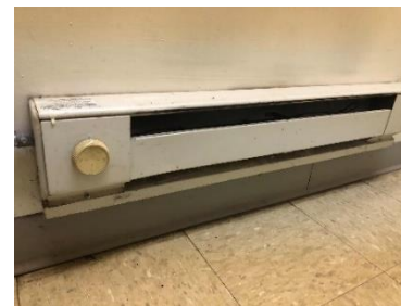
Electric Resistance Heater
