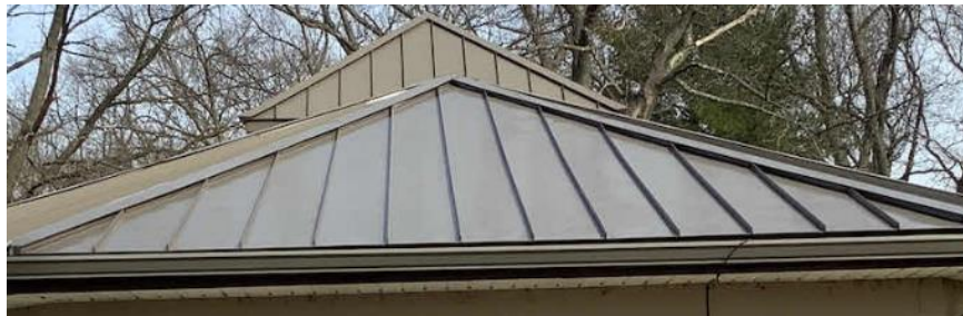
Standing Seam Metal Roof
