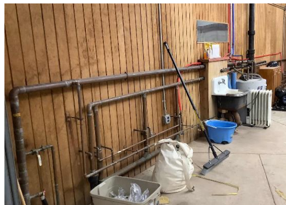
Uninsulated DHW Pipes
