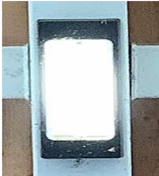
Surface Mounted Metal Halide
