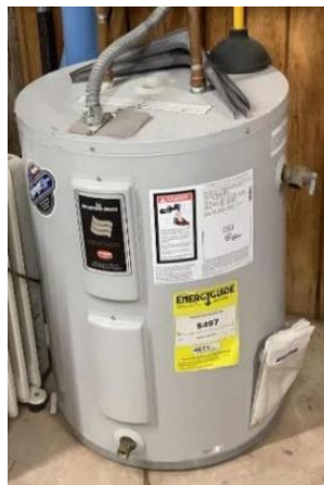
Storage Tank Water Heater
