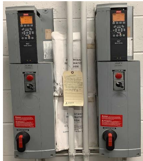
HHW Supply Pump VFDs
