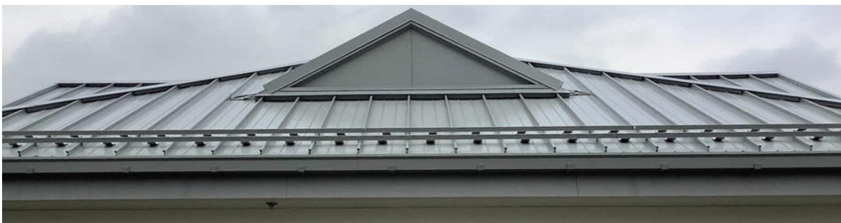
Standing Seam Metal Roof
