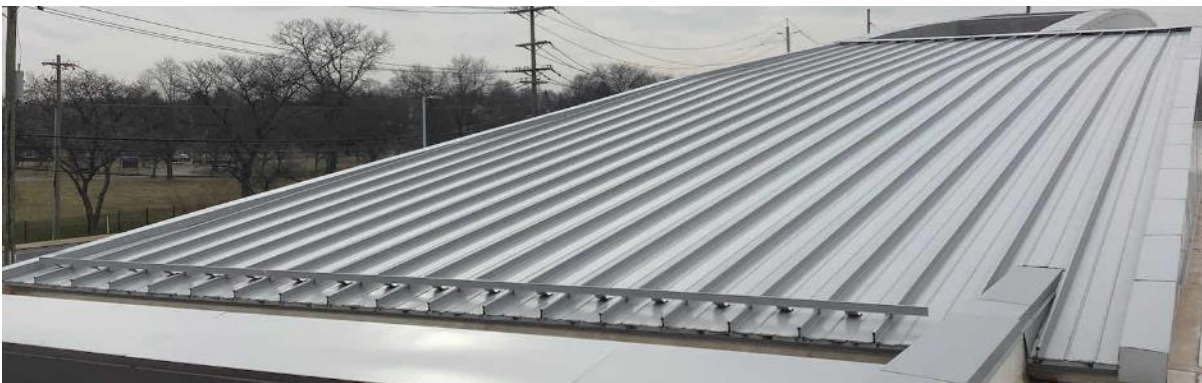
Standing Seam Metal Roof
