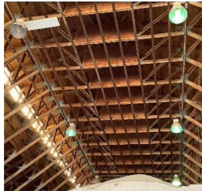
Interior Metal Halide Lighting
