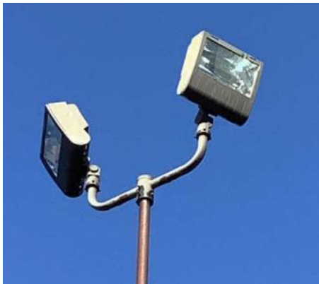
Exterior Pole Mounted HPS
