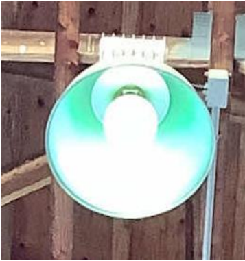
Interior Metal Halide Lighting
