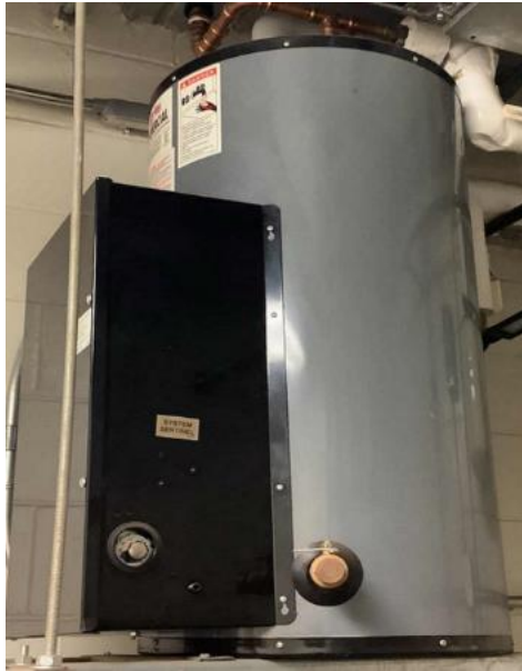
Operations Garage DHW Tank
