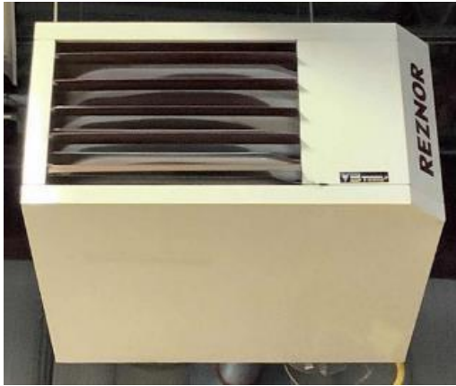
Gas Fired Unit Heater
