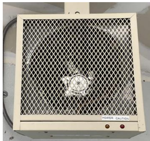
Electric Resistance Unit Heater
