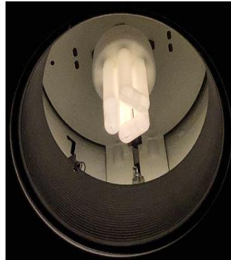
Recessed Can Triple Biaxial CFL Lamp
