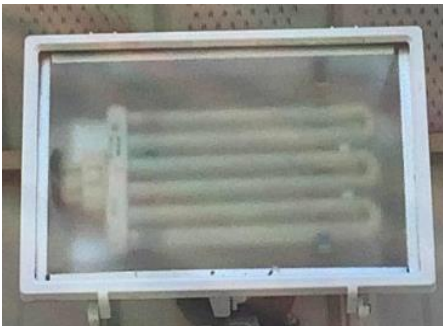
Exterior CFL Floodlight
