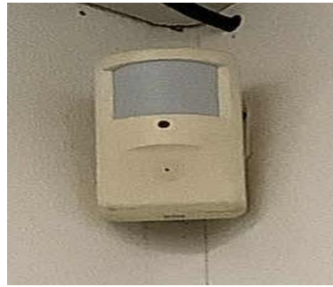
Wall Mounted Occupancy Sensor
