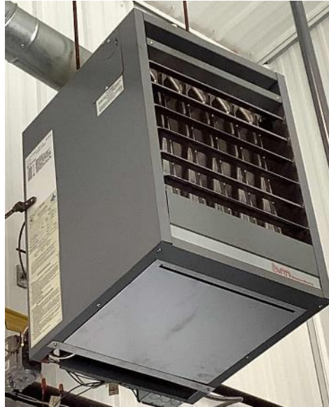
Gas-Fired Unit Heater
