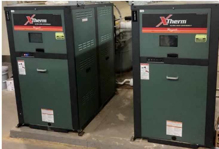
Public Safety Building Condensing Boilers
