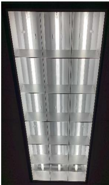
4-Foot Linear Fluorescent Tubes
