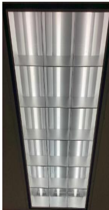
4-Foot Linear Fluorescent Tubes
