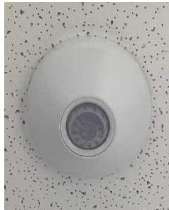
Ceiling Mounted Occupancy Sensor
