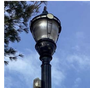
Pole Mounted LED Light
