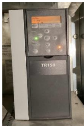
AHU-2 VFD
