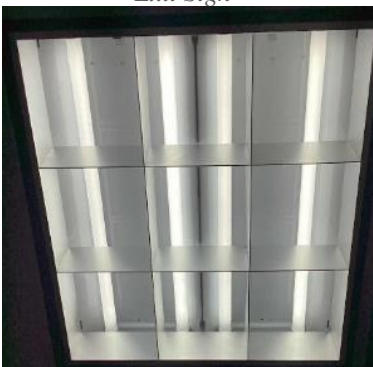
Exit Sign, 2-Foot Linear Fluorescent Tubes
