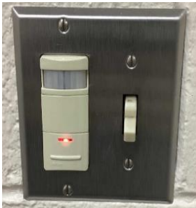
Wall Mounted Occupancy Sensor with Switch
