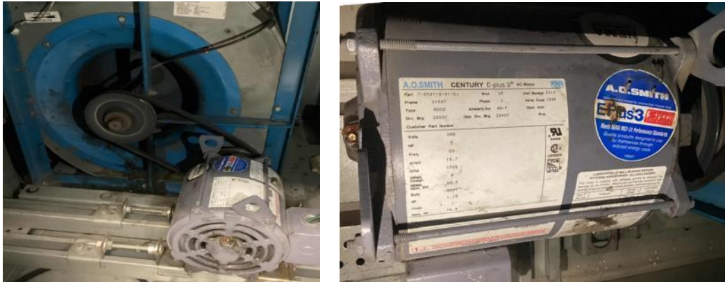
AHU-3 Supply Motor
