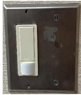
Wall Mounted Occupancy Sensor
