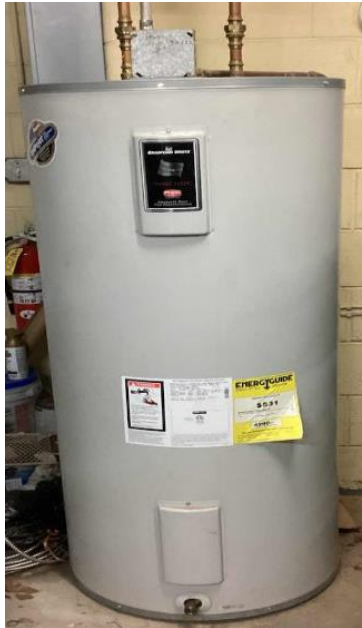
Electric DHW Heater
