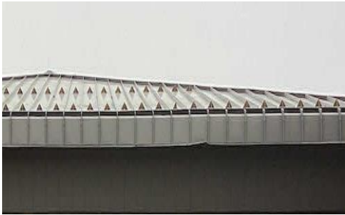
Standing Seam Metal Roof
