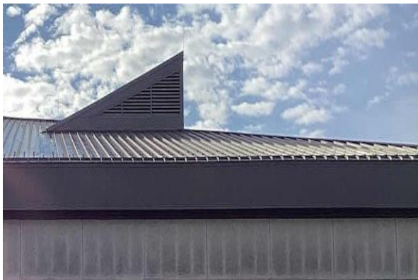
Standing Seam Metal Roof
