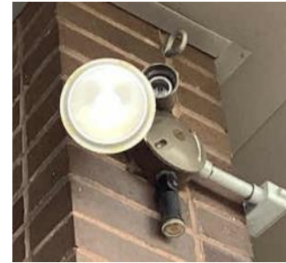
Exterior Recessed Can & LED Spotlight
