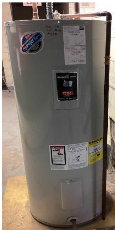
Electric DHW Heater
