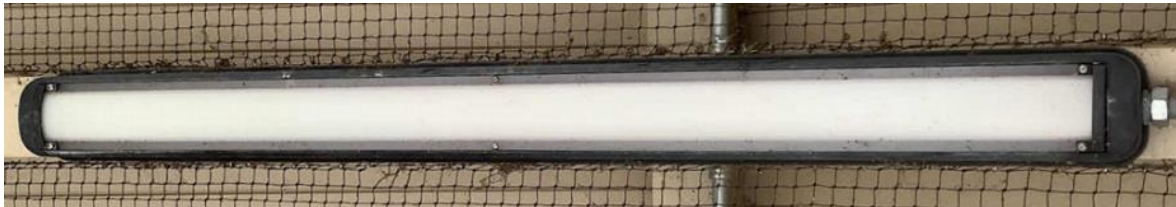
4-Foot Ambient LED Fixture
