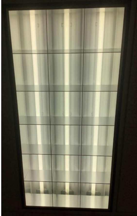
4-Foot T8 Linear Fluorescent Tubes
