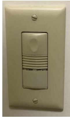
Wall Mounted Occupancy Sensor
