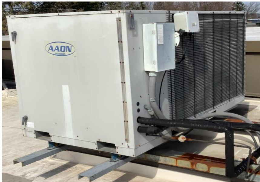
3-Ton AHU Condensing Unit
