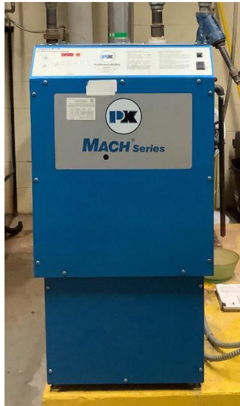
Condensing Heating Hot Water Boiler
