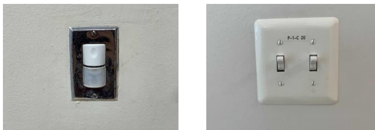
Occupancy Sensor and Wall switches
