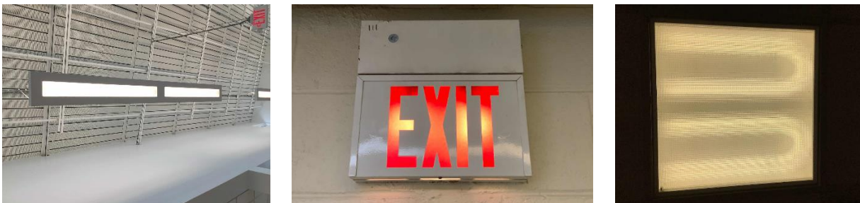
LED Fixtures, CFL Exit Sign, and U-Bend Linear Fluorescent lamps.
