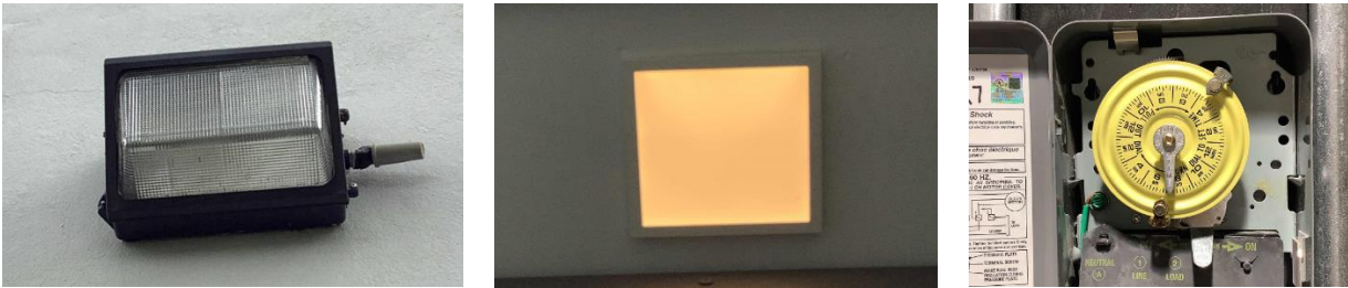
LED Wall Pack, LED Cove Light, and Timer
