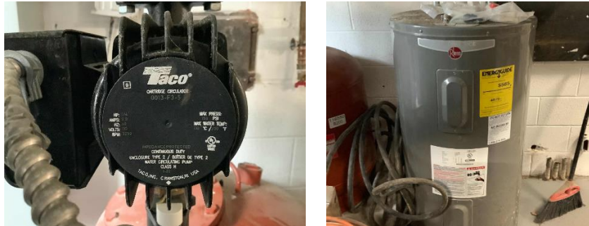
Domestic Hot Water Circulation Pump and Storage Water Heater
