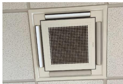
VRV Heat Pumps, Ceiling Mounted Heat Pump Console, And Unit Controls
