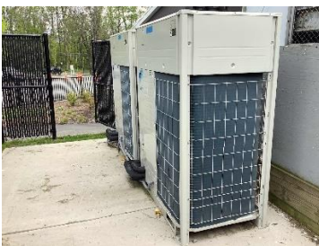
VRV Heat Pumps, Ceiling Mounted Heat Pump Console, And Unit Controls
